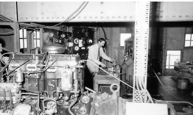
Fig 0.64 Engineer at work in Red Sands Sea Fort during Radio 390 occupation. Photographer: Martin Stevens
