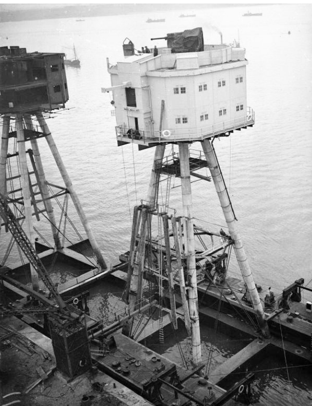
Fig 0.32 1942 Red Sands second generation Army Forts construction.
