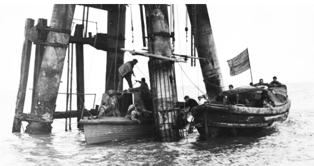
Fig 0.55 Fisherman building cage around damaged structure.
