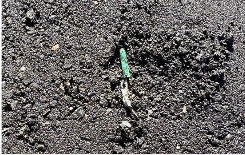
Figure 4-6 Temperature Sensor in the First Lift of the Binder Course
