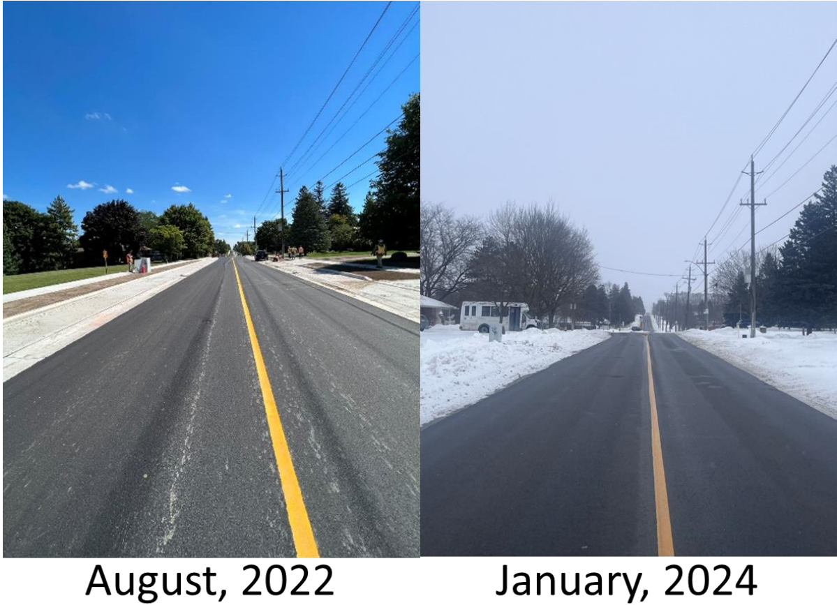
Figure 7-16 Pavement Surface Conditions
