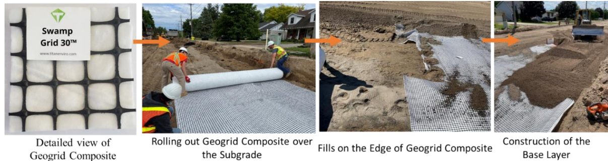
Figure 4-3 Installation of Geogrid Composite on the Subgrade
