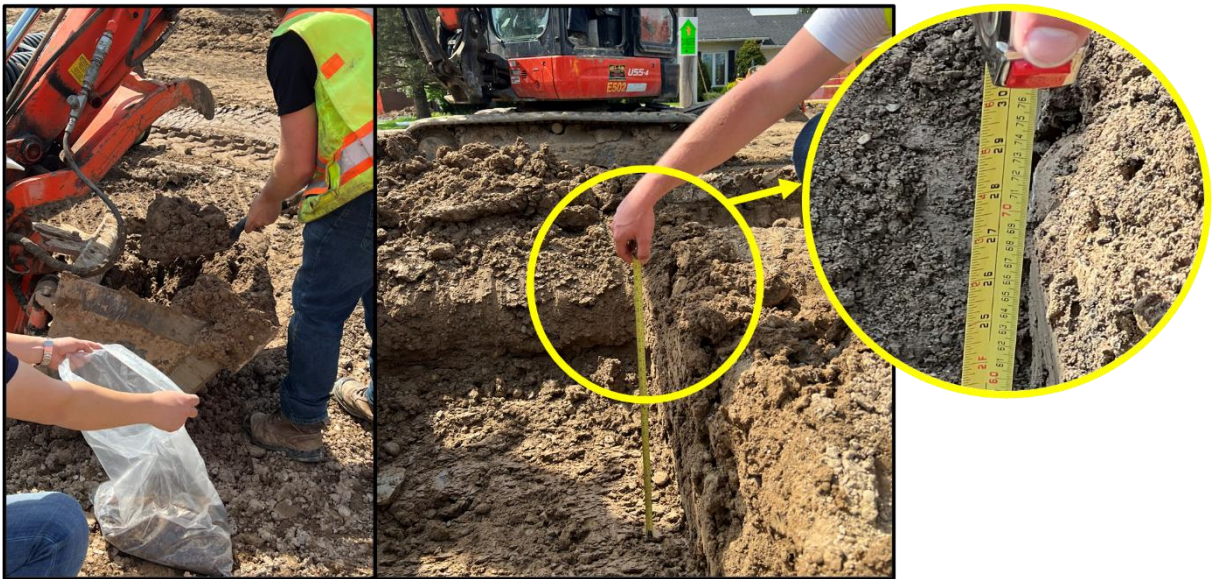
Figure 4-17: Subgrade Sampling from the Field
