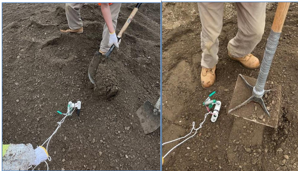
Figure 4-11 Backfilling and Hand Compaction of Granular Base around Sensor Tree
