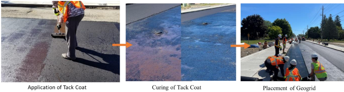
Figure 4-4 Installation of Fibreglass Geogrid in the Asphalt
