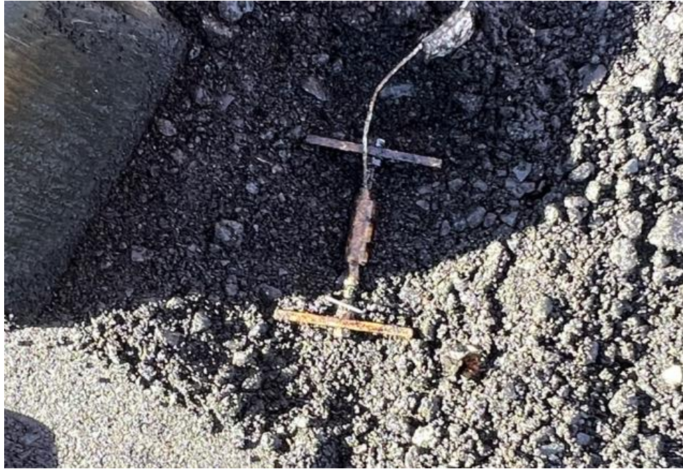
Figure 4-8 Installation of Starin Gauge
