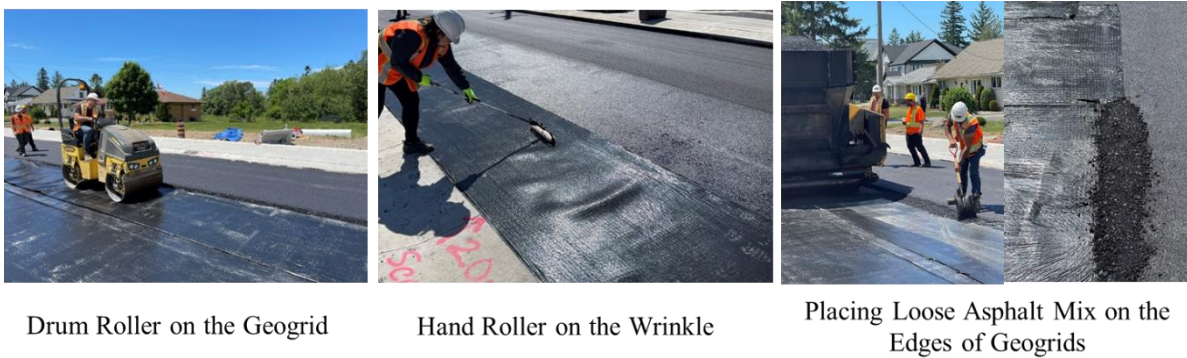
Figure 4-5 Special Measures Taken during Fibreglass Geogrid Installation
