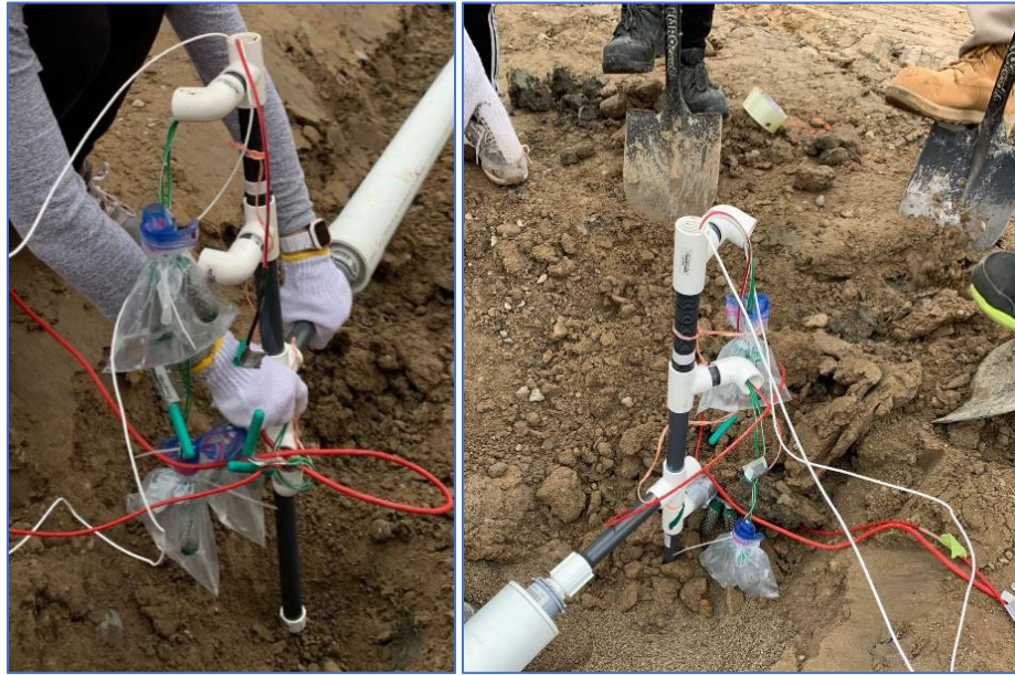
Figure 4-10 Installation of Sensor Tree in the Subgrade
