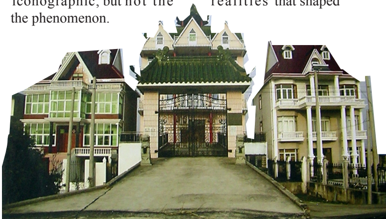
Fig. 1.9 Hybrid Chinese roof on concrete houses.
