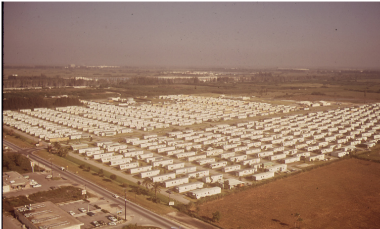
FIGURE 23 Trailer Park Encroaches Upon the Boundaries of the Everglades National Park Trailer parks often neglect urban design elements that help to humanize traditional neighbourhoods. Sidewalks, street lights, front lawns, and social spaces seem to be missing from this example of a trailer park.
