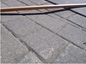
WP063 – Curb cut with protruding concrete.
