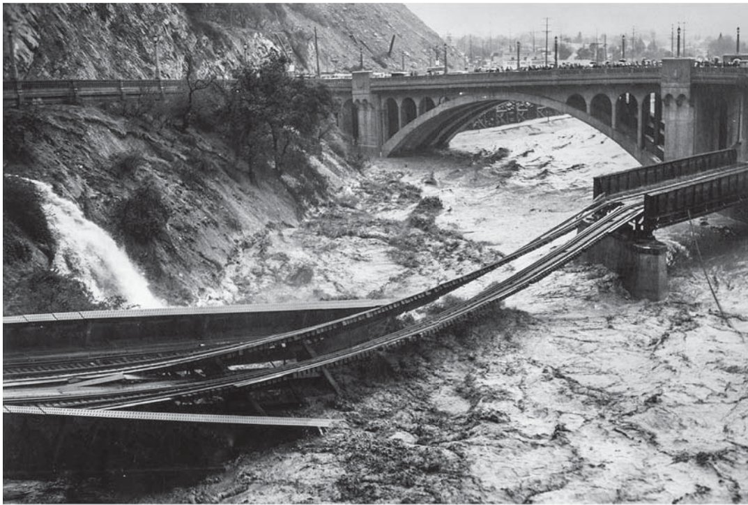
Fig. 1.12 Floodwaters in Los Angeles River destroy Southern Pacific Railroad Bridge at North Figueroa Bridge (March 2, 1938)
