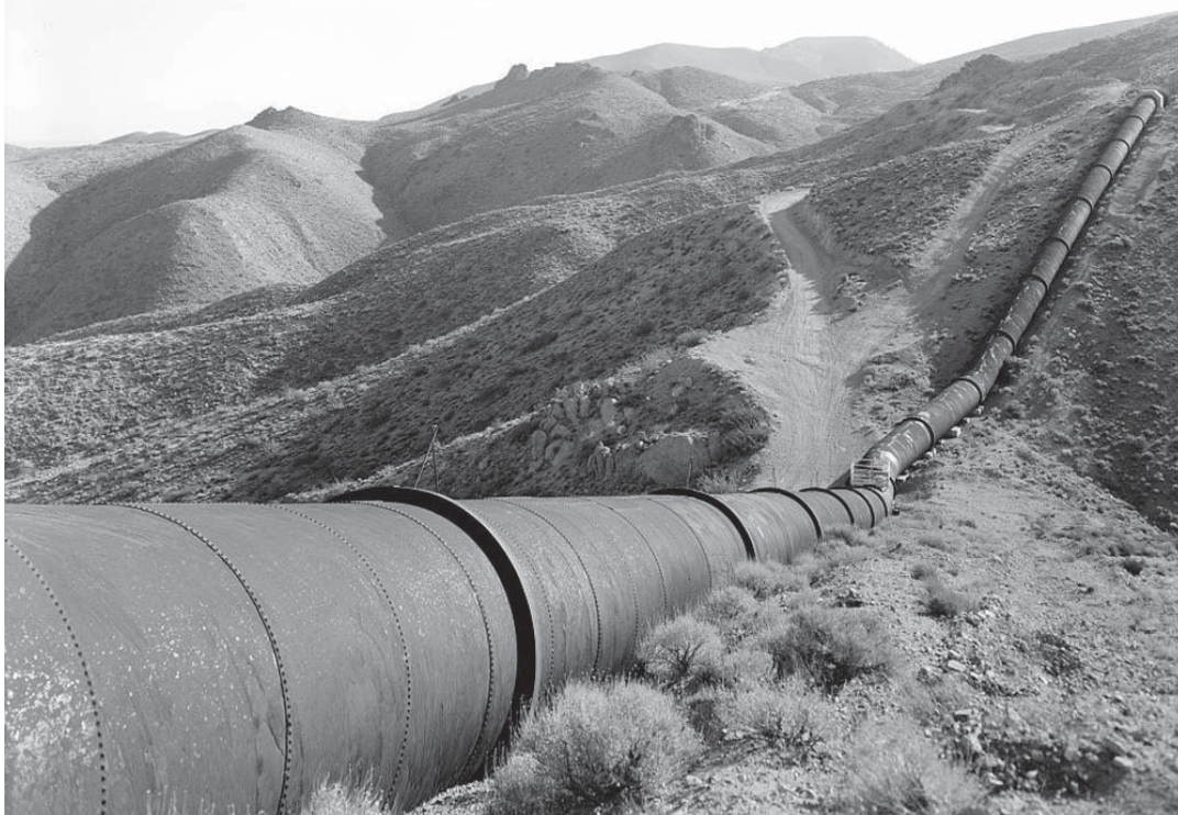
Fig. 1.11 Los Angeles Aqueduct at Jawbone Canyon
