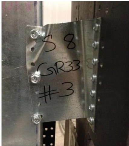
(a) Shear buckling failure
