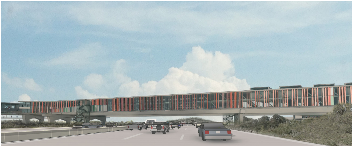
Fig.113-View from the highway on westbound lane, north facade
