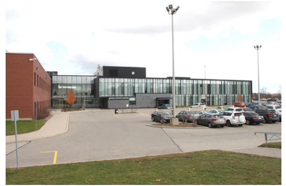
Fig.52-Exterior of Building E & F
