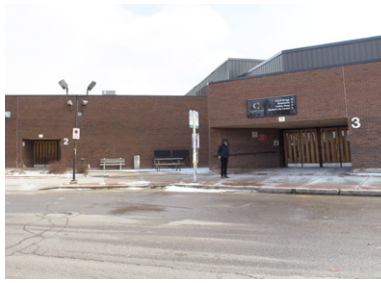
Fig.57-Entrance 2 & 3 to Building A
