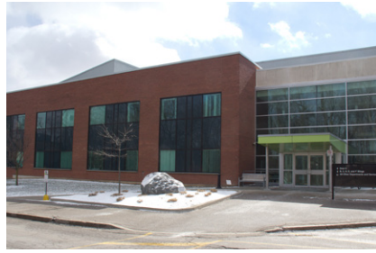
Fig.54-Entrance 6 to Building E
