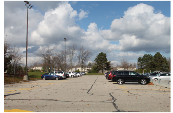
Fig.50-View of the North parking lot
