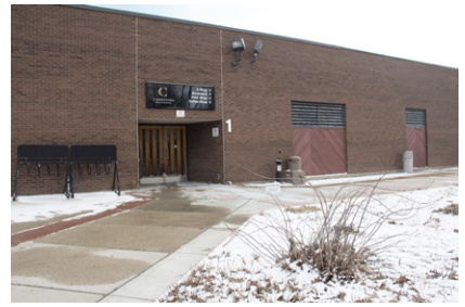
Fig.58-Entrance 1 to Building A
