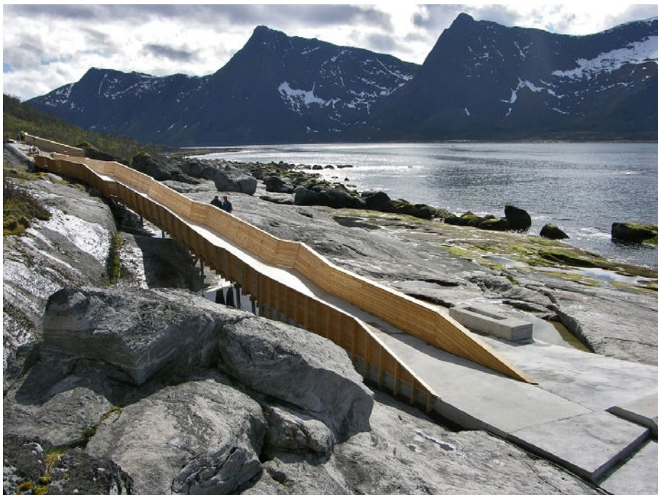
Fig 5.05 Tungeneset rest stop access ramp by Code Arkitektur and Aurora Landskap.
