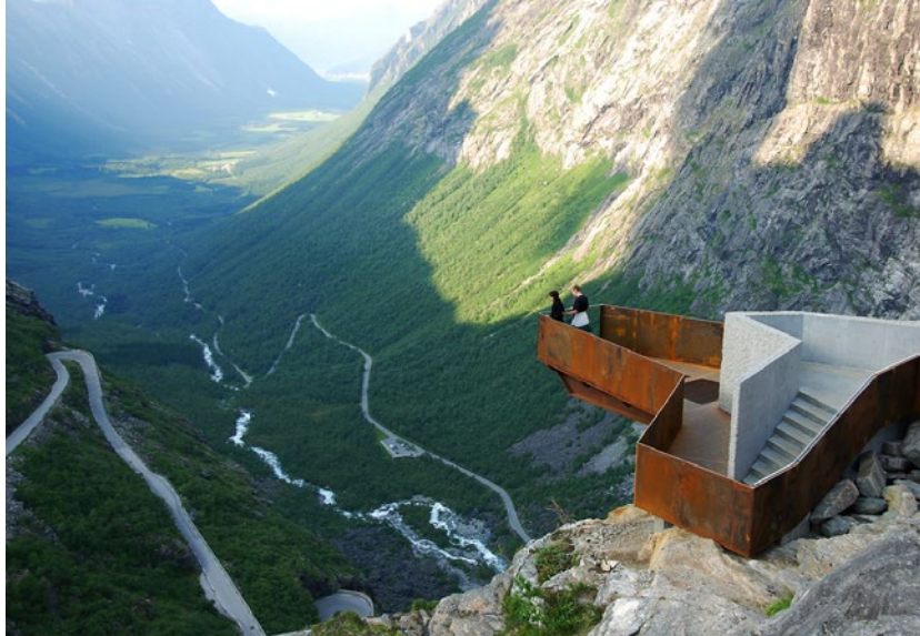
Fig 5.07 Trollstigen viewing platform by Reiulf Ramstad Architects 2.
