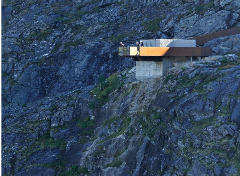
Fig 5.06 Trollstigen viewing platform by Reiulf Ramstad Architects 1.
