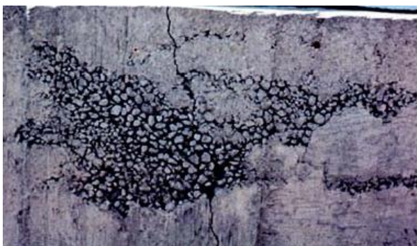
Figure 2-6: Honeycombing (ACI 201.1R-08)
