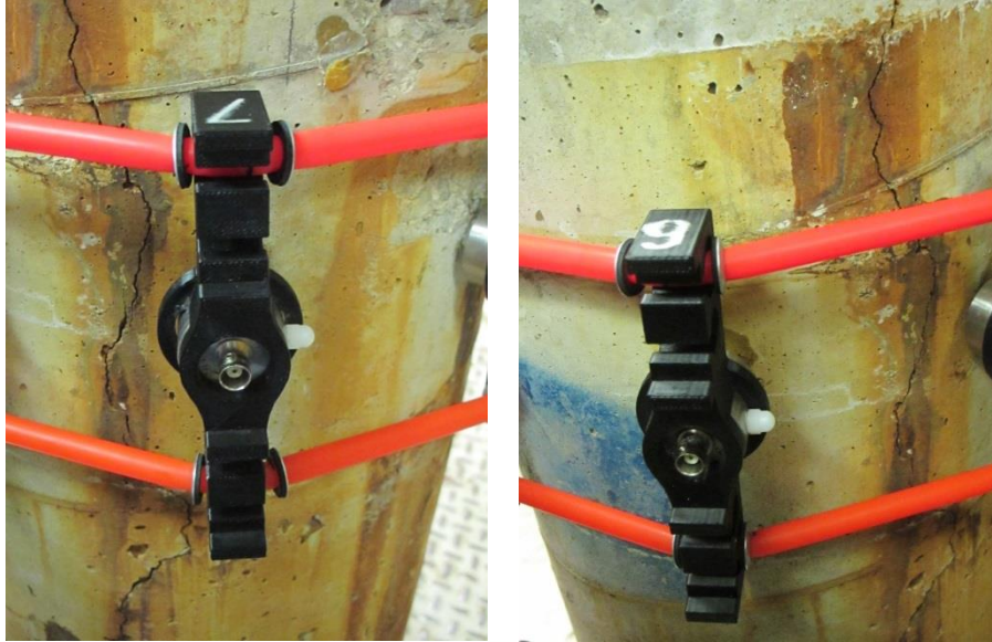
Figure 7-19: Longitudinal cracks caused by the corrosion of the reinforcement
