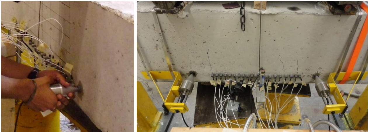
Figure 6-3: Mounting of the source transducers (left: manually, right: rigid frame)
