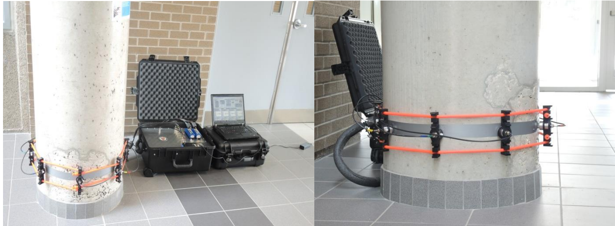
Figure 7-14: Column tested that presents honeycombing
