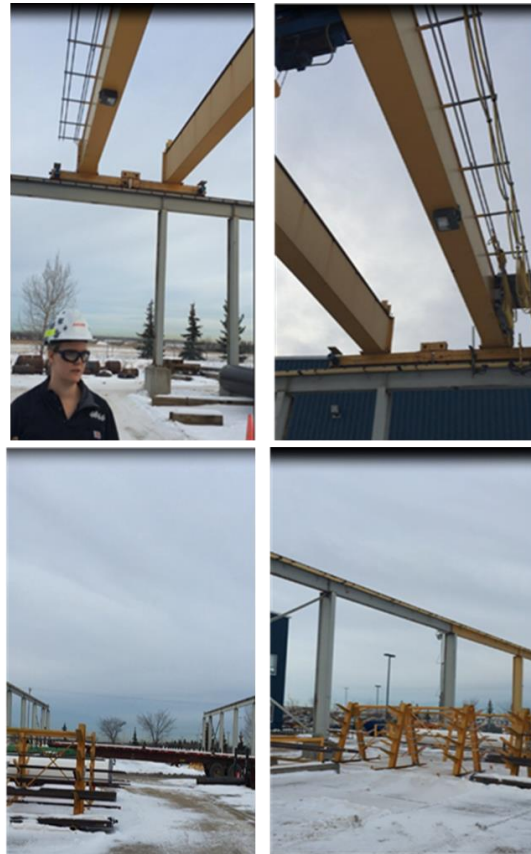
Figure 2-10. Delivered material will be picked by onsite crane and placed on the racks.
