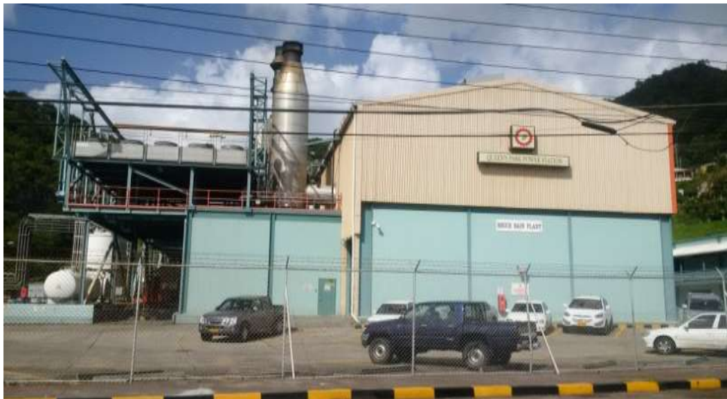
Figure 3.9 Grenlec Power Plant
