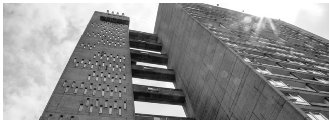
Figure 04.05.b: Balfour Tower, London, by Ernő Goldfinger
