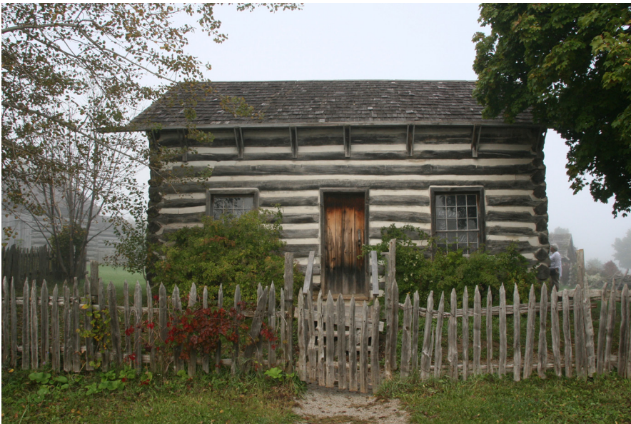
Fig. 1.26 Log cabin vernacular of North American settlers. The use of logs for the exterior walls reflects the abundance of wood found in the region. There are many variations of the log cabin, reflecting the varied cultural backgrounds. (Cassin House, Country Heritage Park, Milton, Ontario)
