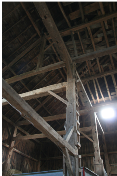
Fig. 2.25 Timber superstructure at the upper floor level of the bank barn.
