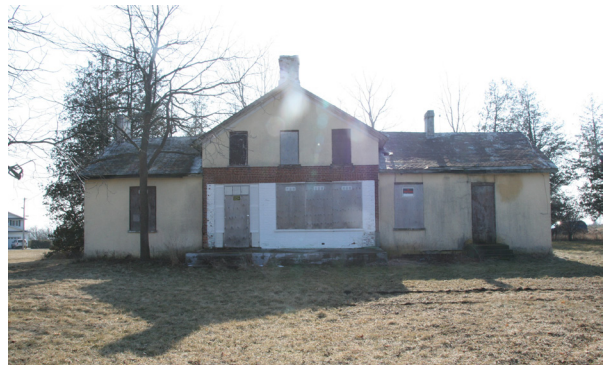
Fig. 2.56 Existing abandoned Lakeview Lodge.
