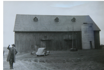
Fig. 2.24 Earlier image of Wilhome Farms bank barn. Built in 1865. Clad in barn board.
