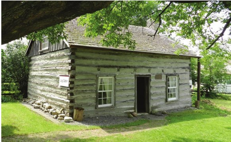
Fig. 2.8 Log cabin at Ameliasburgh Heritage Village. Built in 1860, the cabin was moved to the village in 1969 and was fully restored in 2016.
