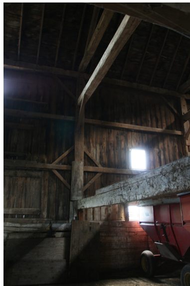
Fig. 2.25 Timber superstructure at the upper floor level of the bank barn.
