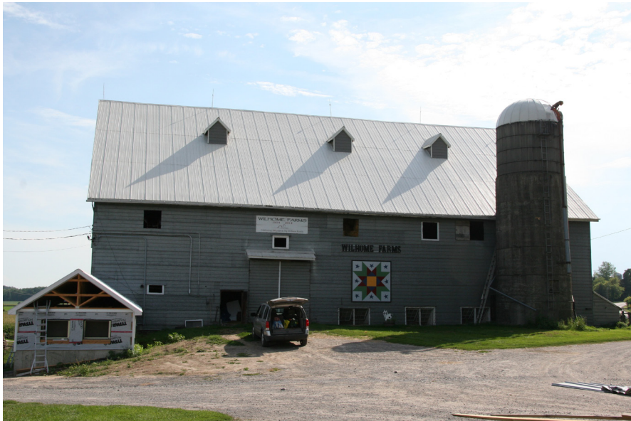
Fig. 2.23 Wilhome Farms bank barn, 2017. Clad over with aluminum siding.
