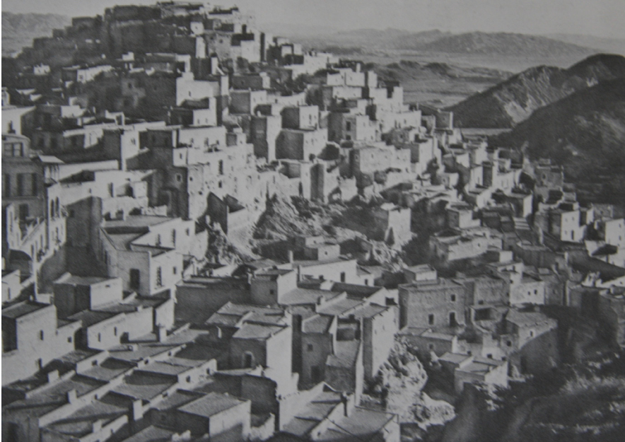
Fig. 1.25 Hill town vernacular featured in Architecture without Architects exhibition. Mojacar, located on the coast of Spain. The arid climate dictates the use of thermal mass that absorbs heat during the day and releases it at night. Small windows limit heat gain from the sun and white-washed exterior and interior walls reflect light. Passive strategies for heating, cooling and lighting through material use and building design.
