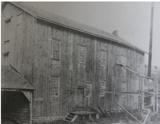
Fig. 2.9 Clapp's Upper Mill, later known as Scott's Mill, located in Milford. Built in 1845 as part of a milling complex.
