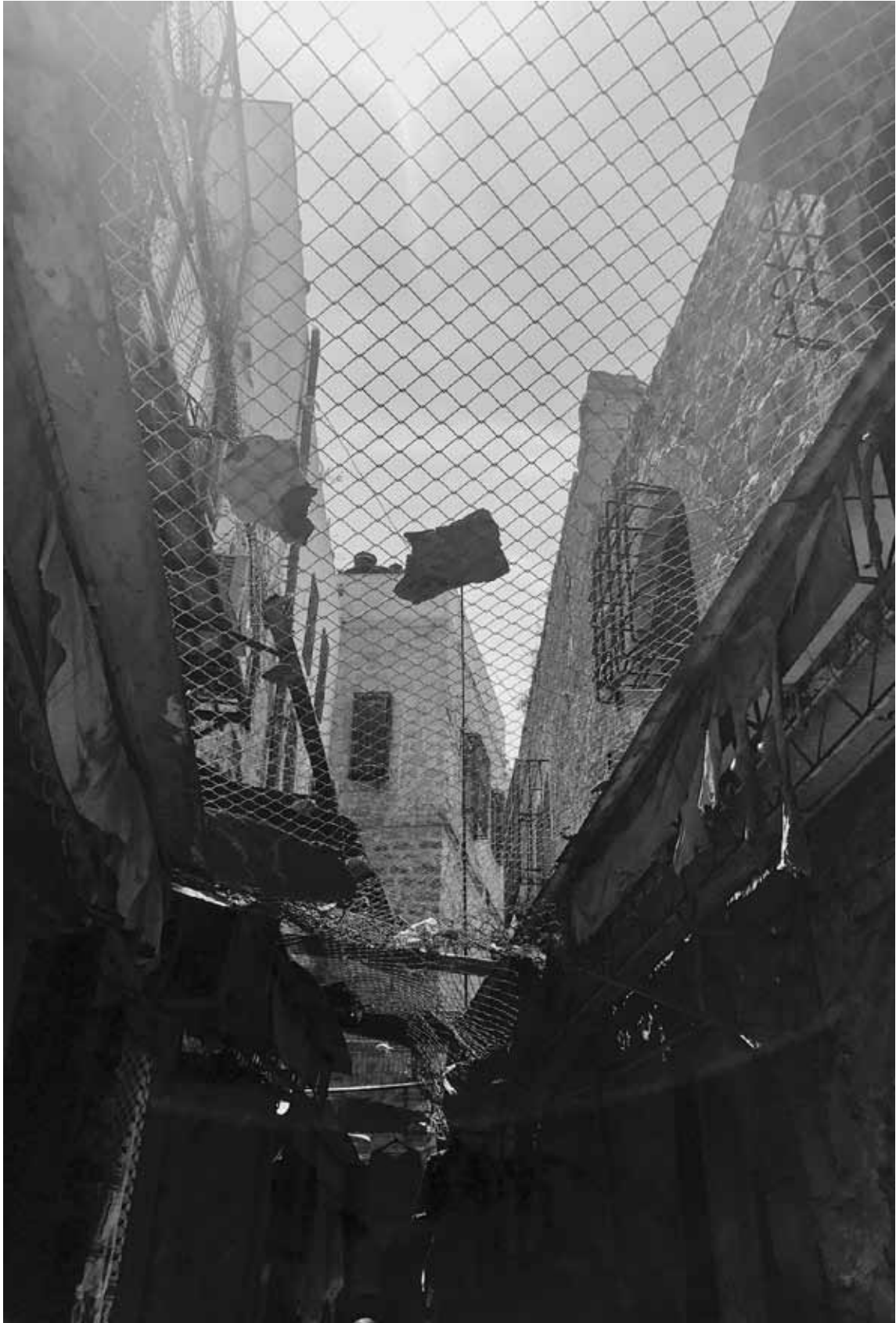
40 Wire grids cover the alleyways of the Market and protect Palestinians passing by from trash thrown down by Jewish settlers living in the upper storeys. Hebron Old City. The West Bank. May 2017
