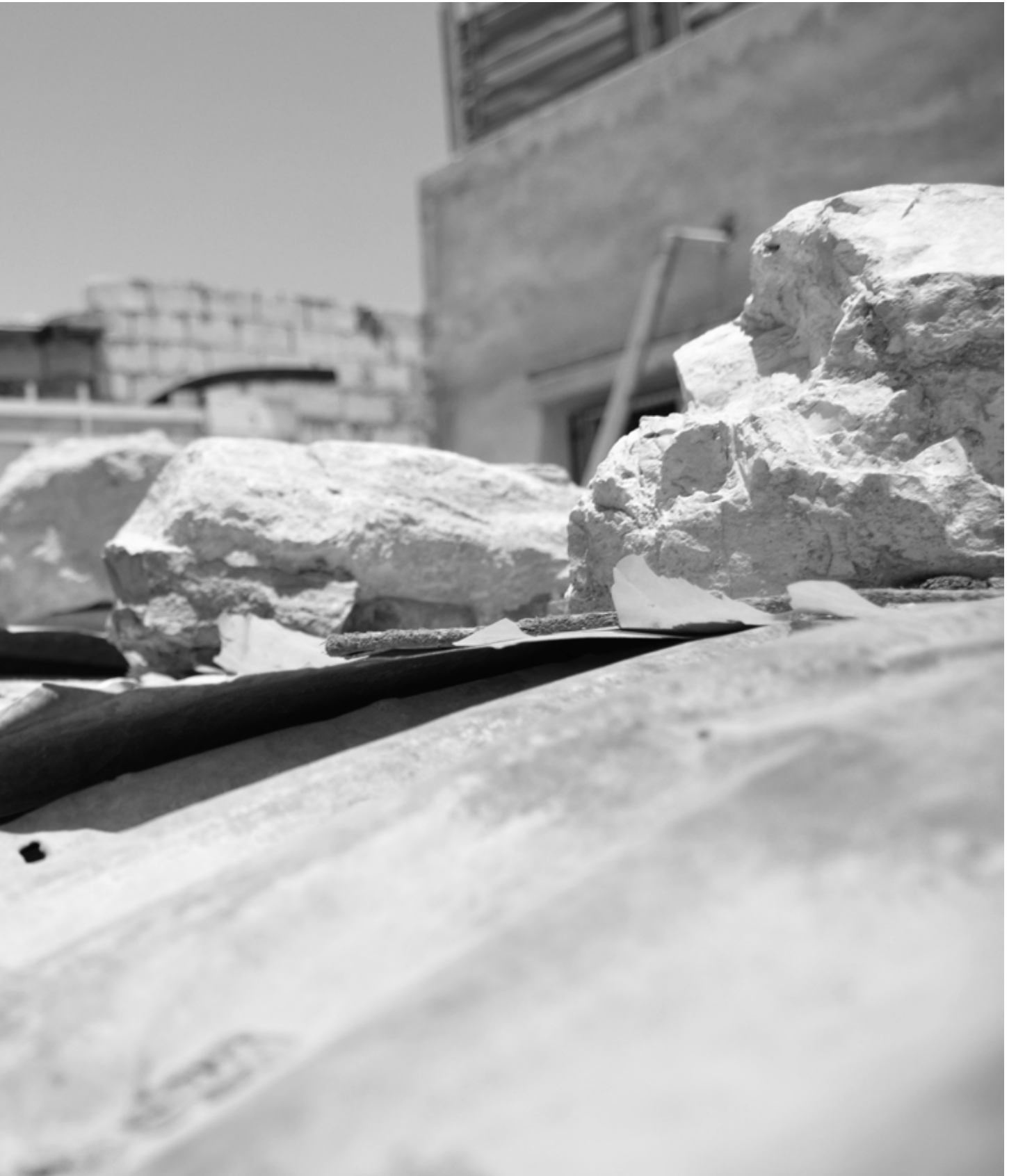
12 Zinc Roof. Marka (Hittin) Refugee Camp, Amman, Jordan. June 2017
