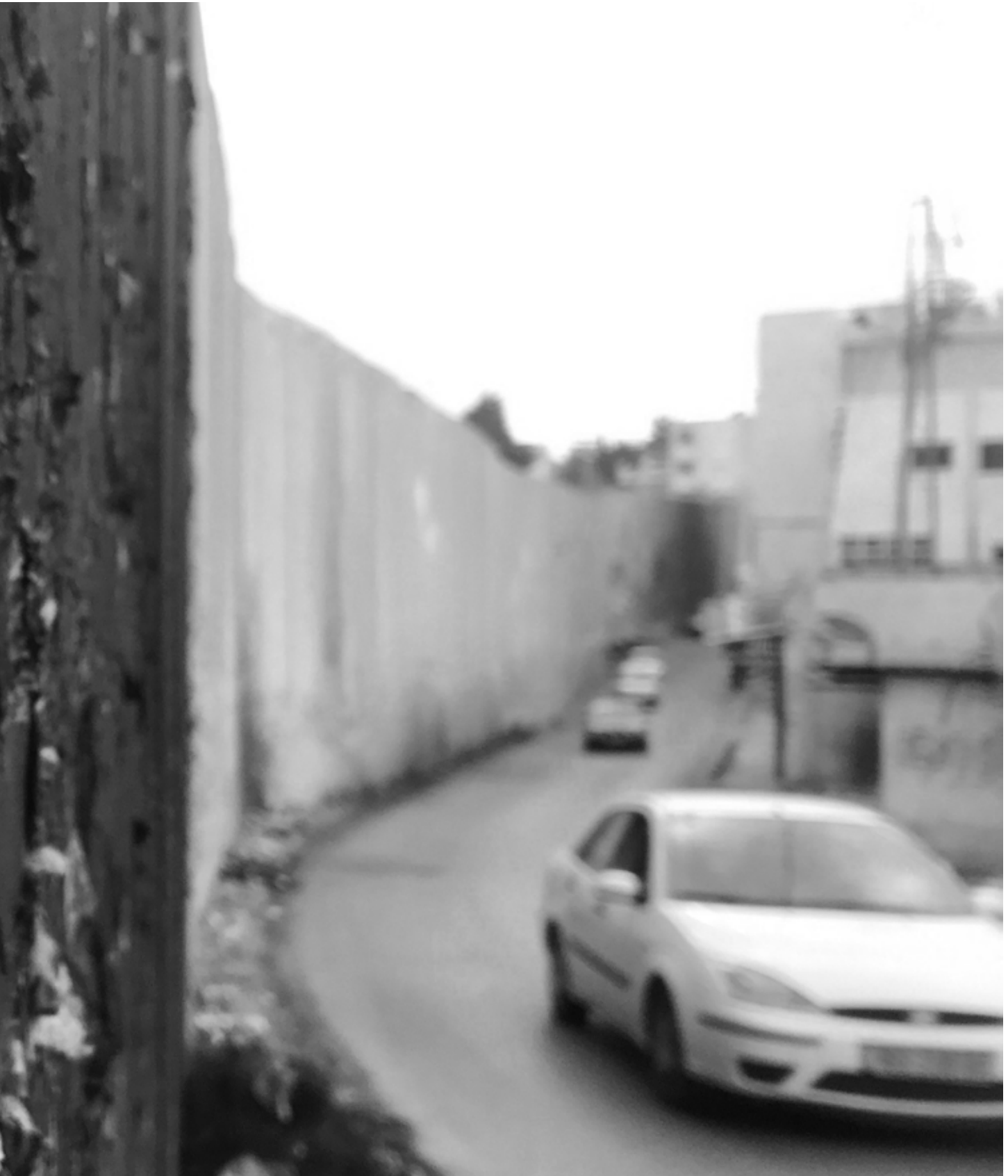
67 The West Bank Wall. Abu Dis, The West Bank May 2017
