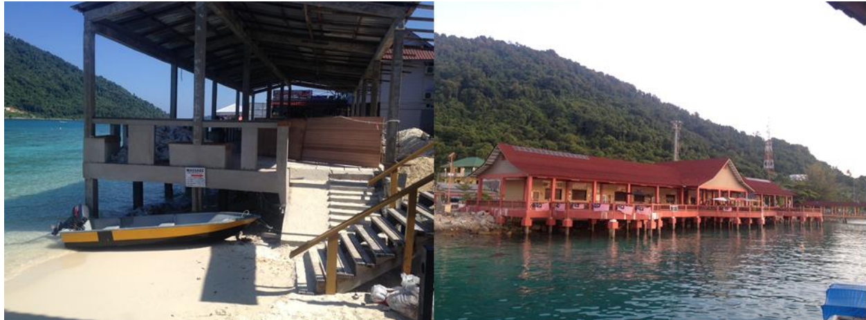
Figure 4.2 – Buildings on shore
