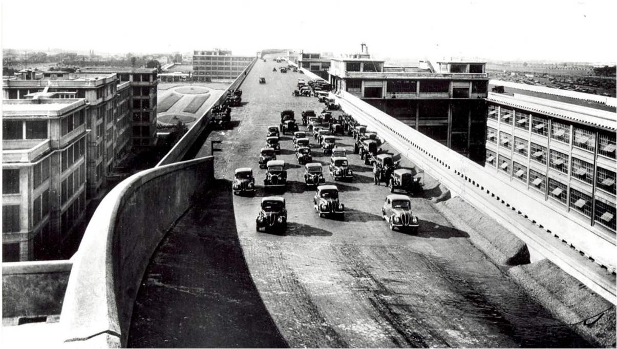
Figure 1.16 - Test track on the roof of the Lingotto Factory
