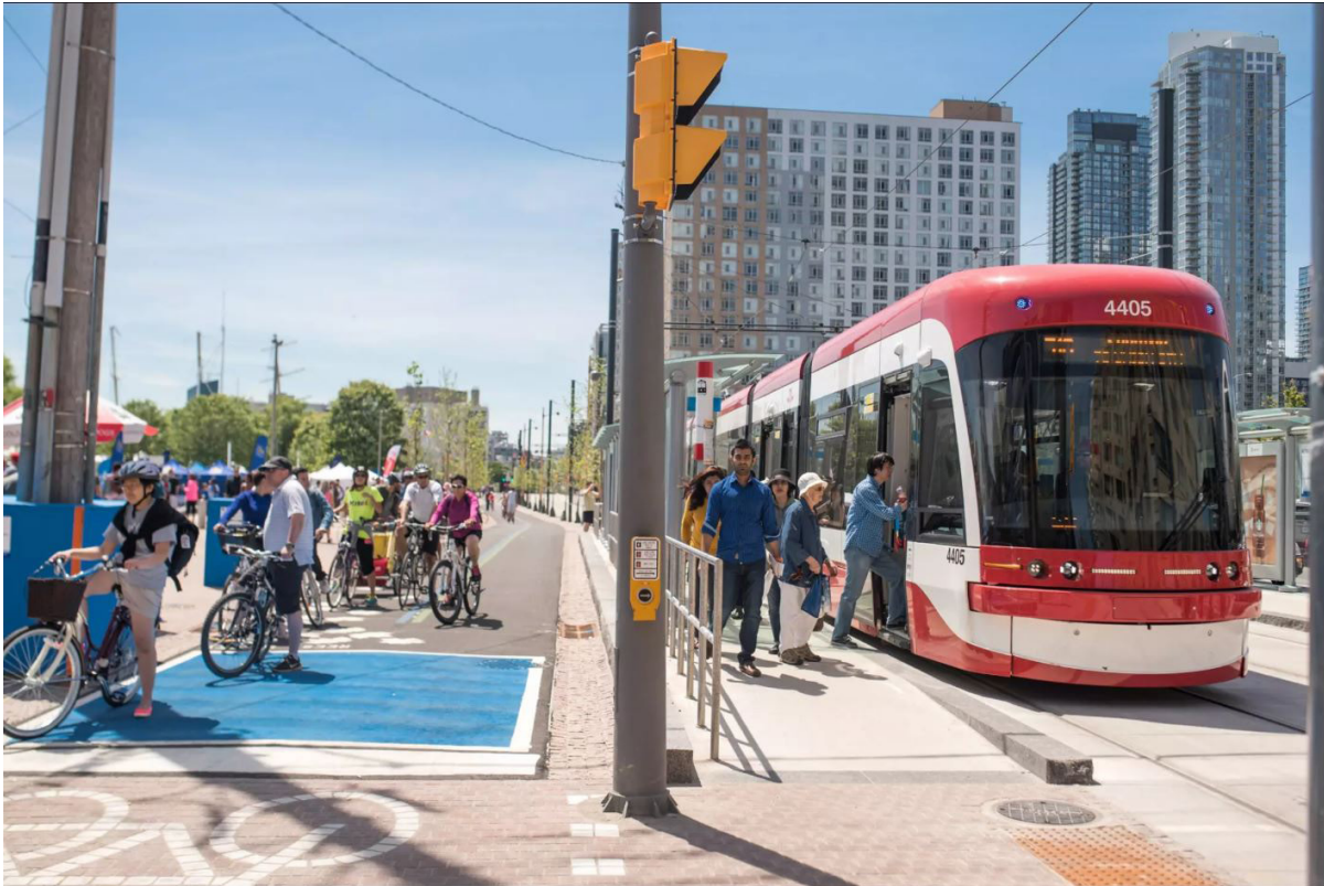
Figure 2.13 - Separate bike lanes and streetcar traffic on Queens Quay
