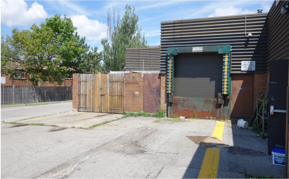
Figure 5.11 - Rear loading dock for the retail plaza
