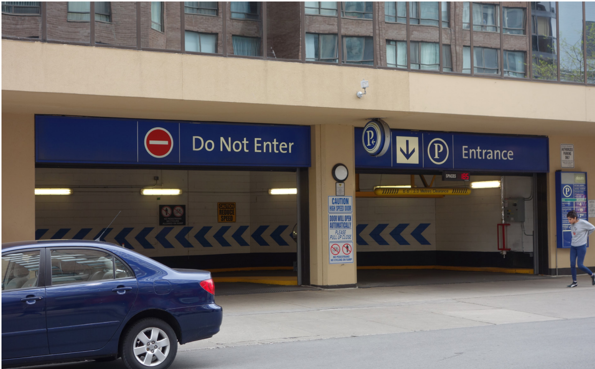
Figure 5.102 - Entrance to the underground public parking lot
