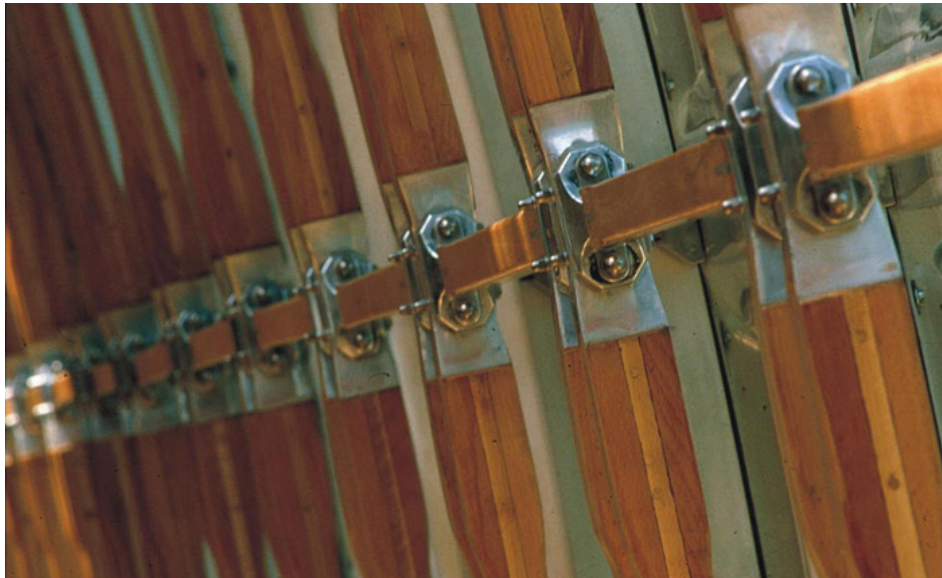
Figure 3.13 IBM Traveling Pavilion. View of junctions in the interior of the pavilion.
