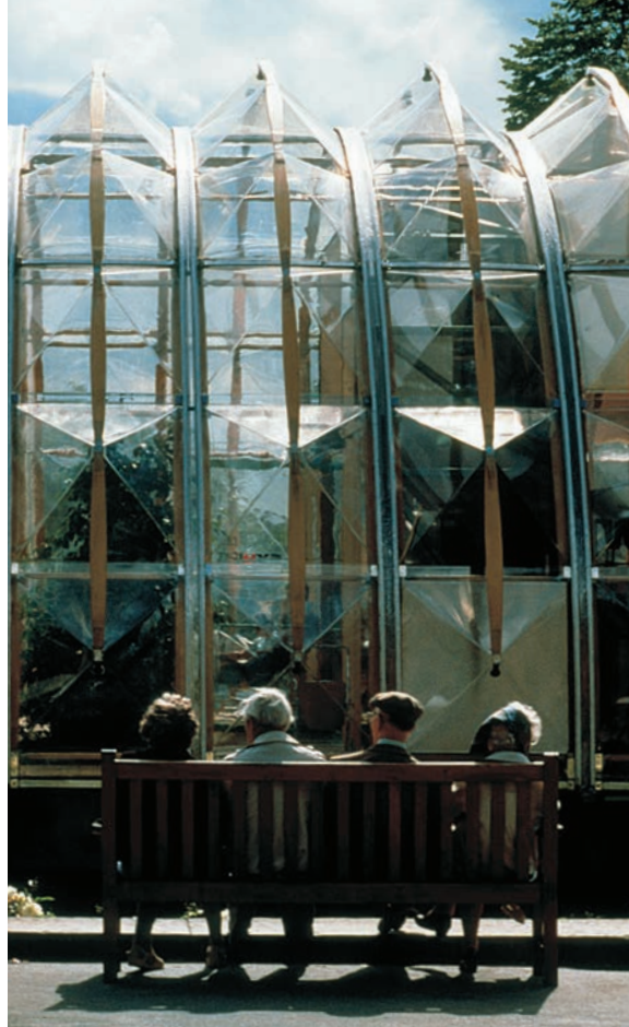
Figure 3.12 IBM Traveling Pavilion. Close-up view of the structure in York suggesting how the public felt with its un-intimidating and welcoming presence.
