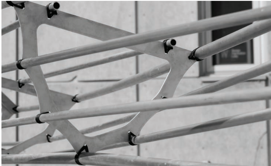
Figure 2.33 Rails to section connection. Connection of the aluminum tubes to the aluminum sections.
