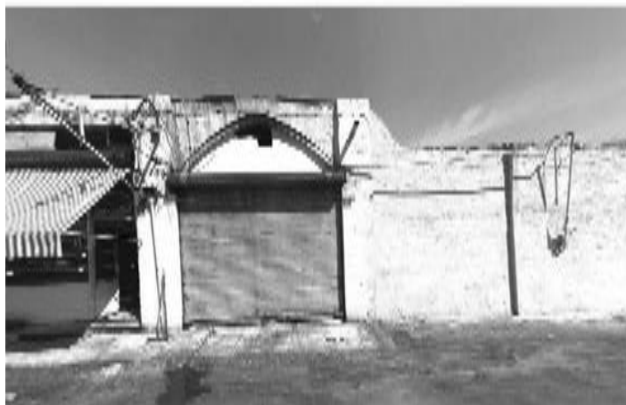
Figure 34. Photos of the old fabric of the potential site – Parking lot
