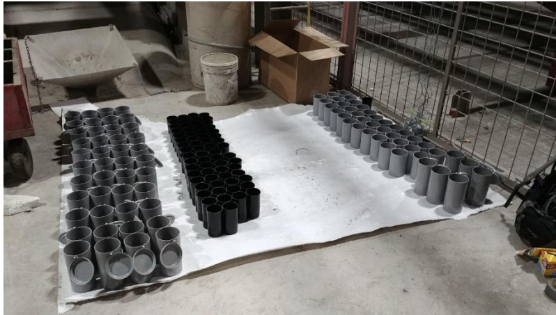
Figure 3.18: Photo of Cylinder Moulds Used for Cylinder Cast (CC) Before Concrete was Placed
