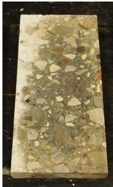
Figure 3.3: Air Void System Sample After Analysis
