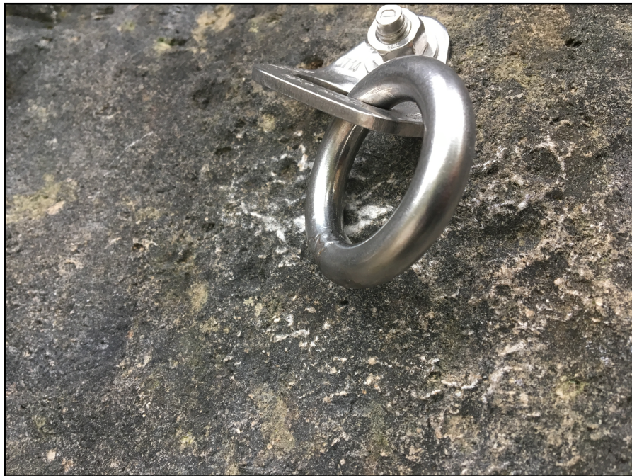
Figure 2. Bolt hanger with ring. This is part of a teaching anchor.
