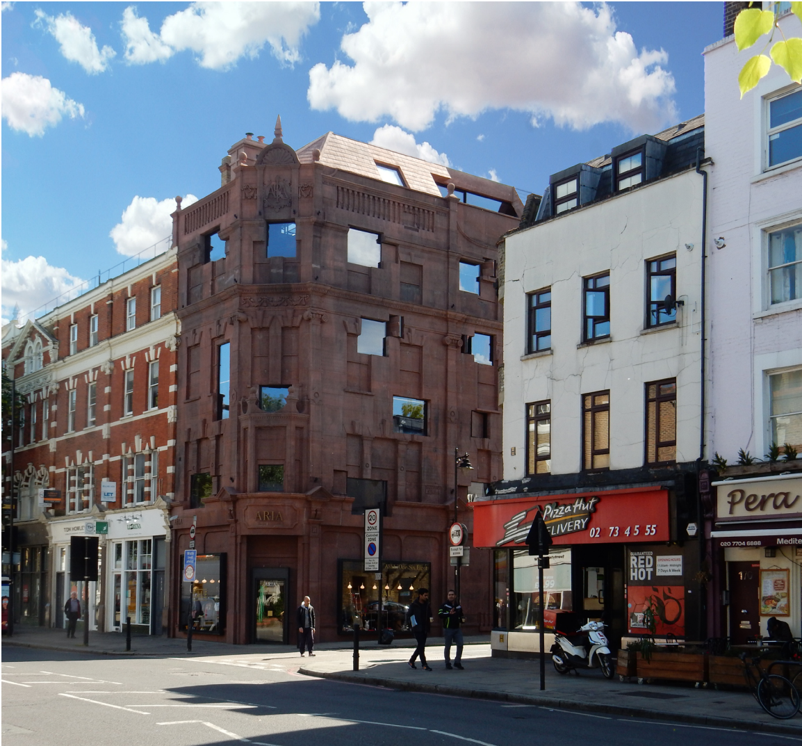
Fig. 7.9) 168 Upper Street in London by Groupwork + Amin Taha Architects (built 2017)
