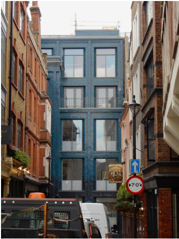
Fig. 2.15) Damien Hirst Headquarters in London (built 2018)
