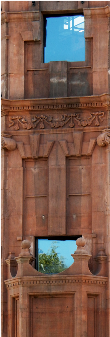
Fig. 7.10) Detail view of 168 Upper Street
