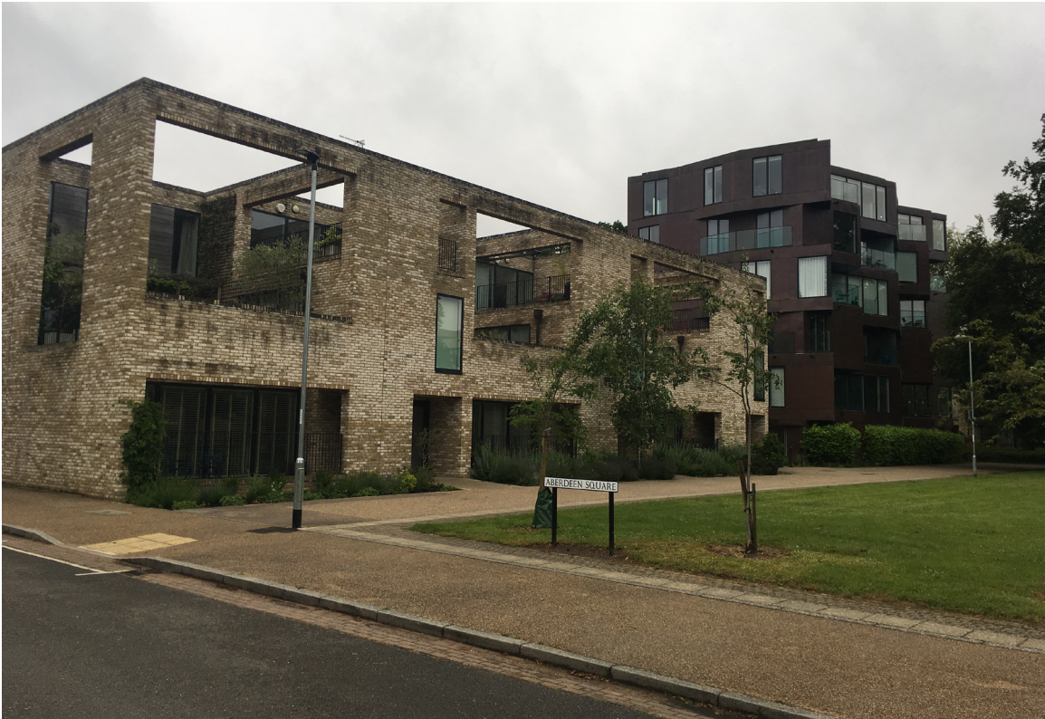
Fig. 3.8) Accordia Housing Development brick and brass buildings
