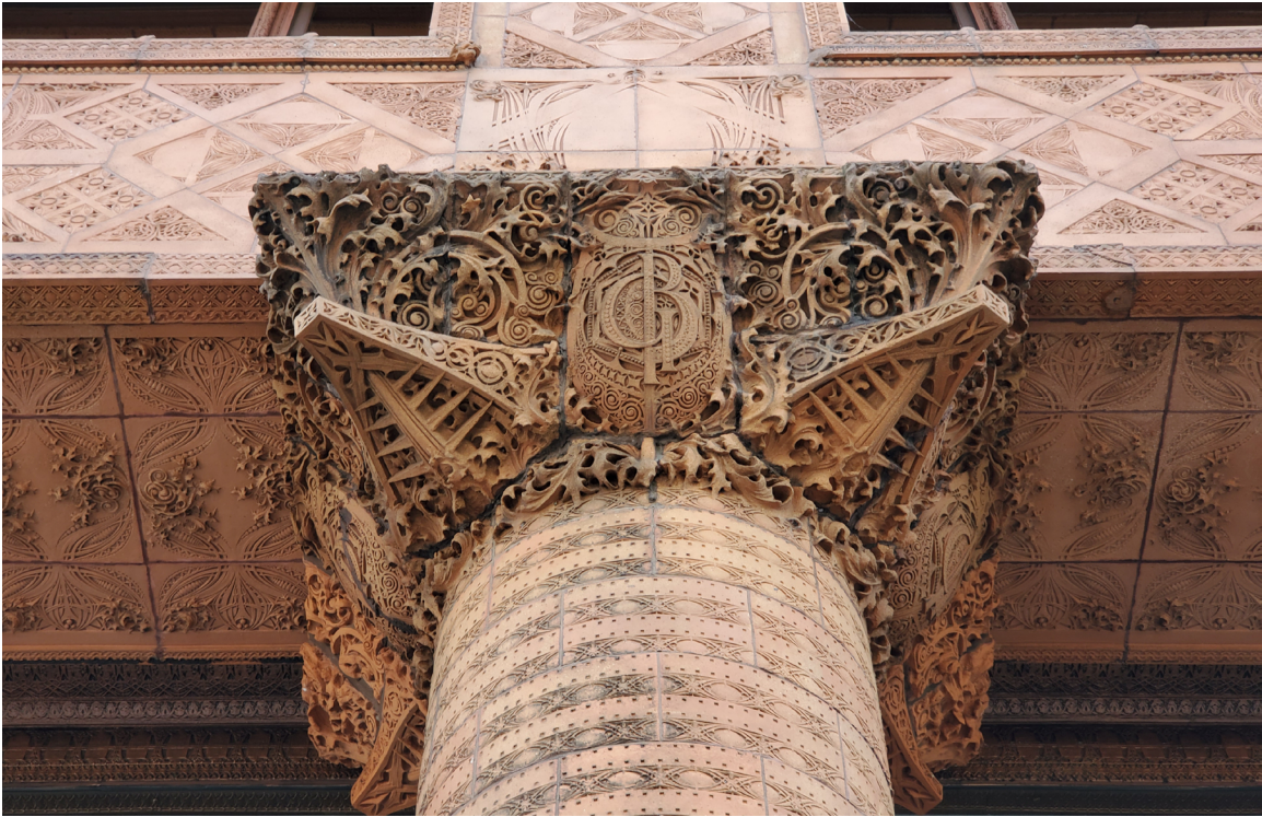
Fig. 6.3) Detail view of the Guaranty building in Buffalo by Louis Sullivan (built 1896)
