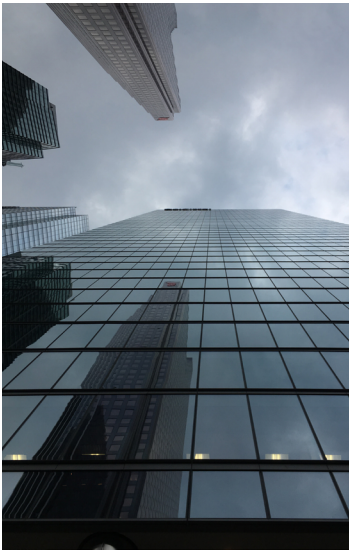
Fig. 4.9) Bay Adelaide Centre in Toronto by KPMB Architects (built 2016)
