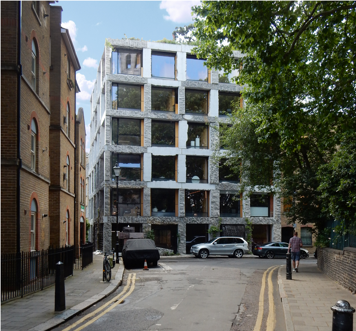
Fig. 7.6) 15 Clerkenwell Close in London by Groupwork + Amin Taha Architects (built 2017)
