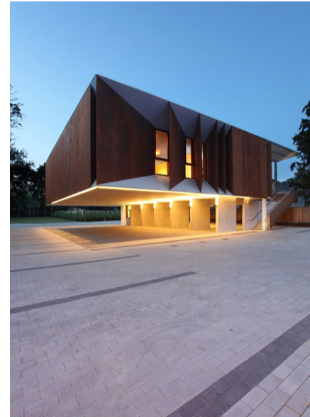
Figure 2.44 The Wong Dai Sin Temple and the parking on site
