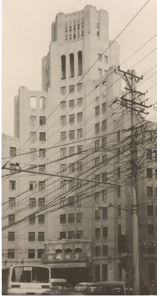
Figure 2.1 The Metropole Hotel in Shanghai Concession, 1933-1934
