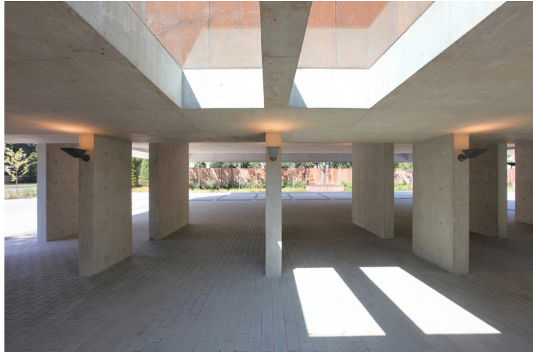
Figure 2.45 Sheer walls supporting the main building & skylights on the terrace
