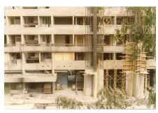
Fig. 5.3 Buttressing of C type building. 1987
