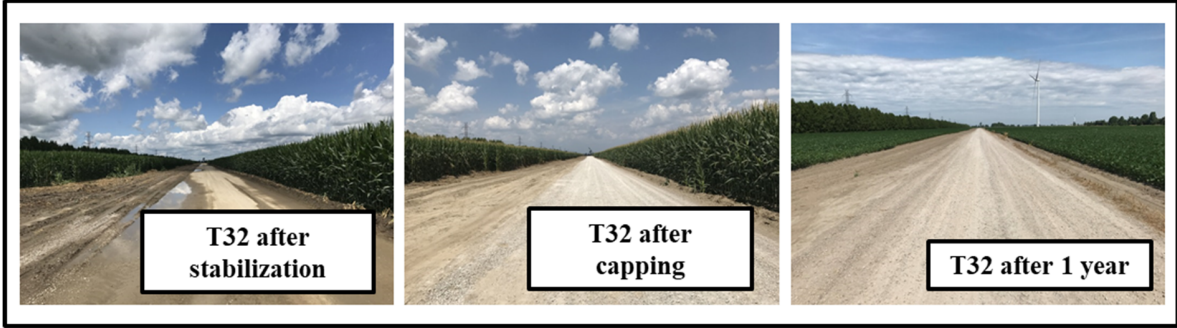
Figure 6-7 Road conditions: T32
