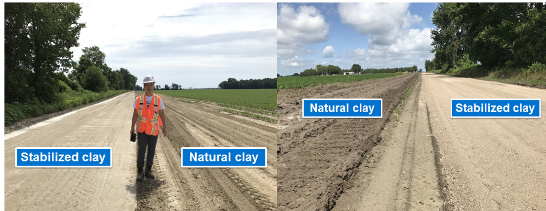
Figure 2-12 Comparison between natural and stabilized clay subgrade (Pictures were taken in Chatham-Kent, 2017).
