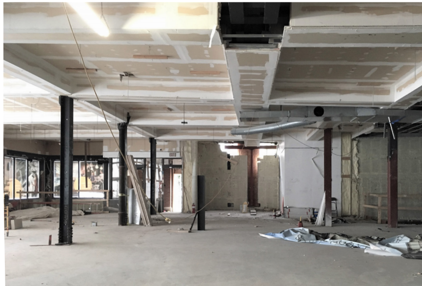
FIGURE 4.09 Interior view - June 27, 2018. Source: Author
