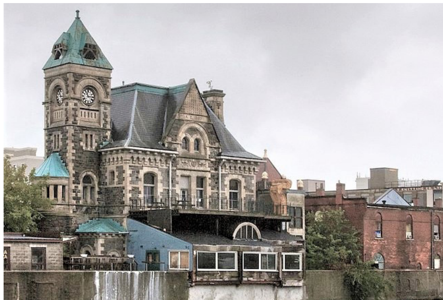
FIGURE 2.06 Abandoned Post Office - 2014. Source: https://commons.wikimedia.org/wiki/File:Galt_Old_Post_Office.jpg
