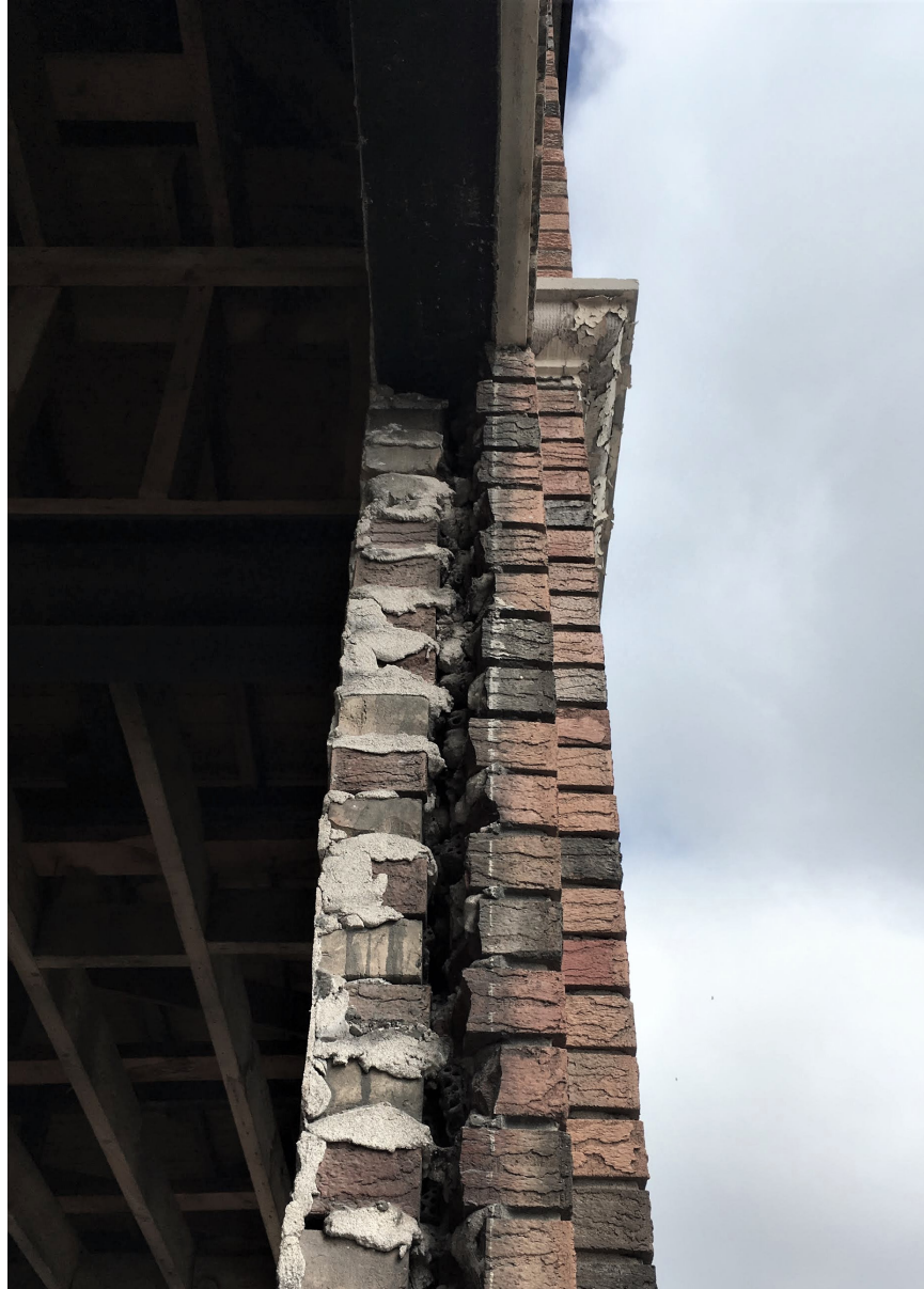
FIGURE 4.10 Exterior wall assembly - September 18, 2018. Source: Author
