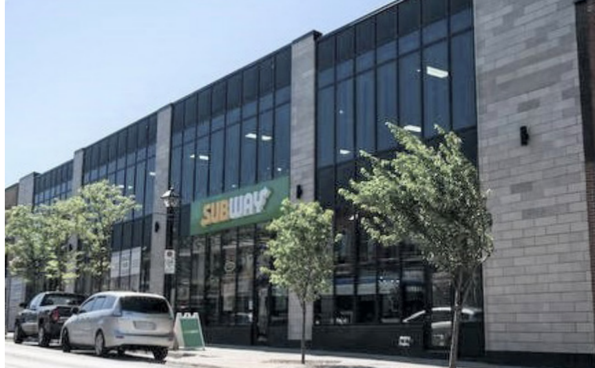
FIGURE 2.25 New facade - 2016. Source: Rego Realty
