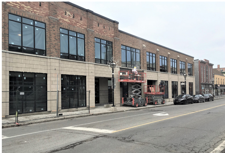
FIGURE 4.15 Windows installed - November 29, 2018. Source: Author
