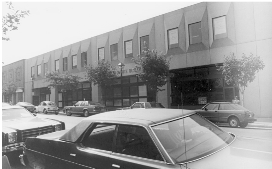
FIGURE 2.24 Arthur White Building - 1984. Source: City of Cambridge Archives
