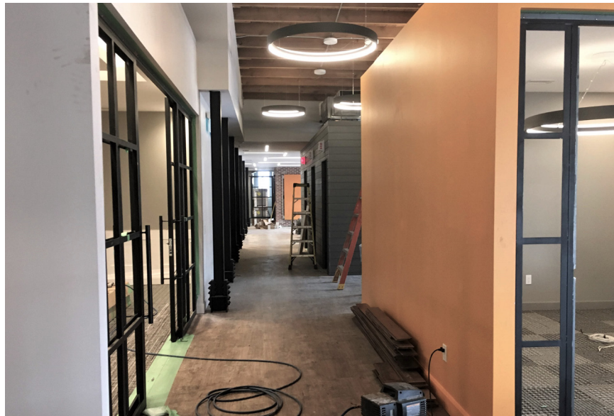
FIGURE 4.20 Second floor finishes - May 2, 2019. Source: Author
