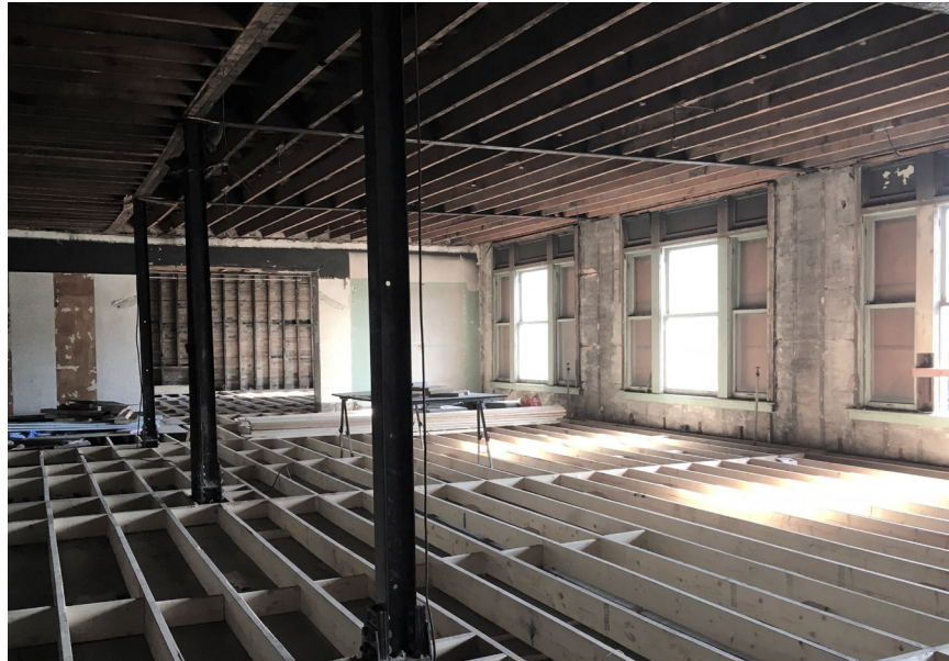
FIGURE 4.06 Leveling the second floor - May 30, 2018. Source: Author
