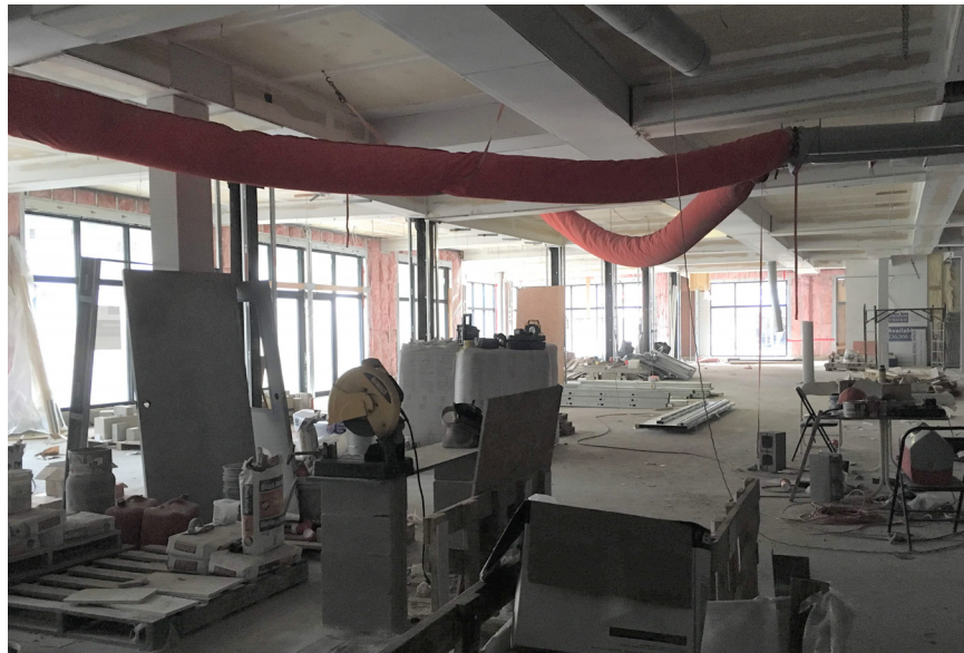
FIGURE 4.16 Main floor - December 19, 2018. Source: Author
