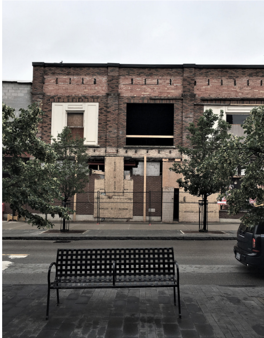
FIGURE 4.08 Moving a column - June 27, 2018. Source: Author
