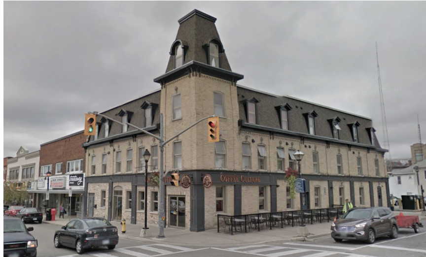
FIGURE 2.20 Facade restoration - 2015. Source: Google Street View
