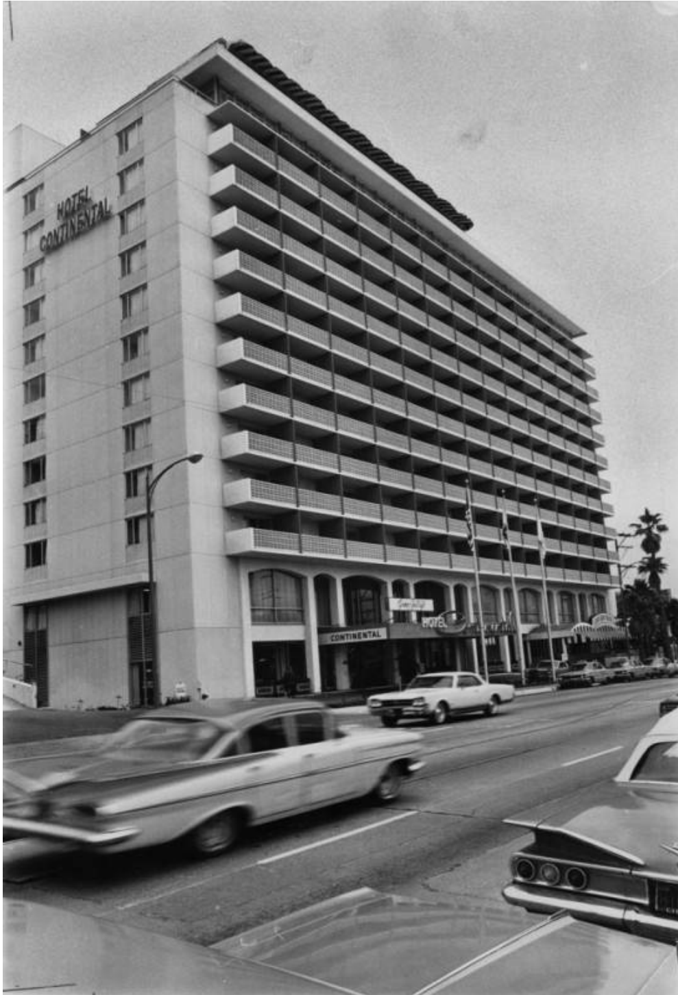
Figure 5.10: At fourteen stories high, The Continental Hyatt House is located at 8401 Sunset Boulevard. Photo dated: January 9, 1966. Retrieved from the Herald Examiner Collection/Los Angeles Public Library.
