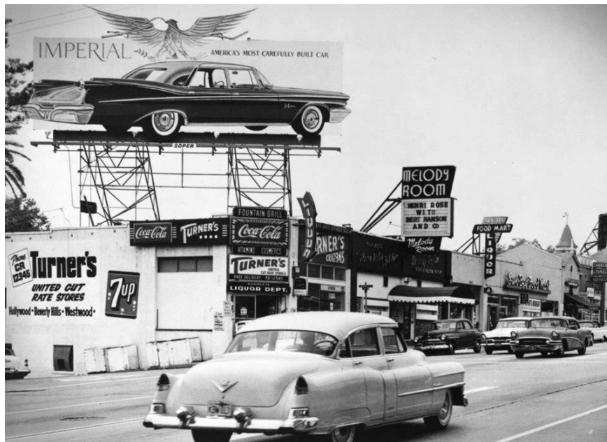
Figure 1.1: A photograph of 8852 Sunset Boulevard as the Melody Room, located to the right of Turner’s Liquor, 1956. Retrieved from Los Angeles Past.
