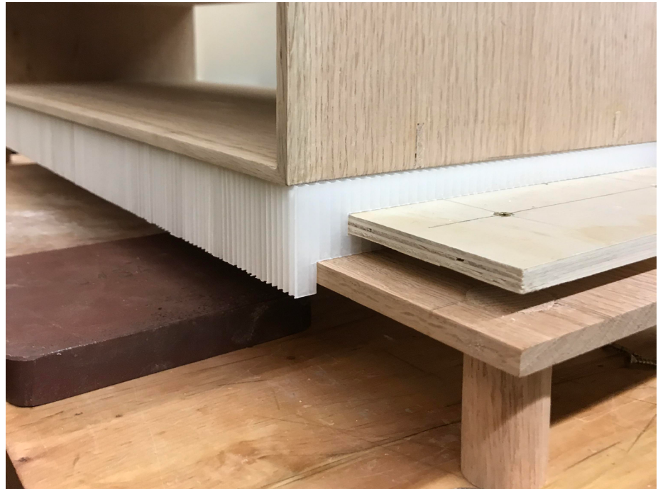
5.28 FuwaFuwa Series: Detail - Wood to corrugated Plastics
