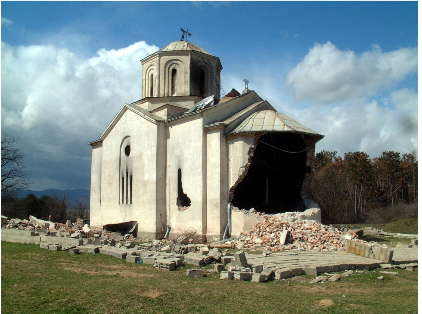
Fig 23. Church of St. Elijah in Podujevo after destruction - 2004
