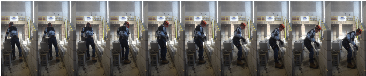
Figure 2-3: A complete CMU lift sequence from pick up to lay down
