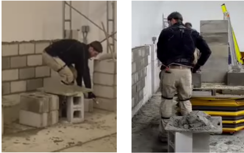
Figure 7-8: Postural differences: picking up a CMU manually (left) and with the self-leveling pallet (right)
