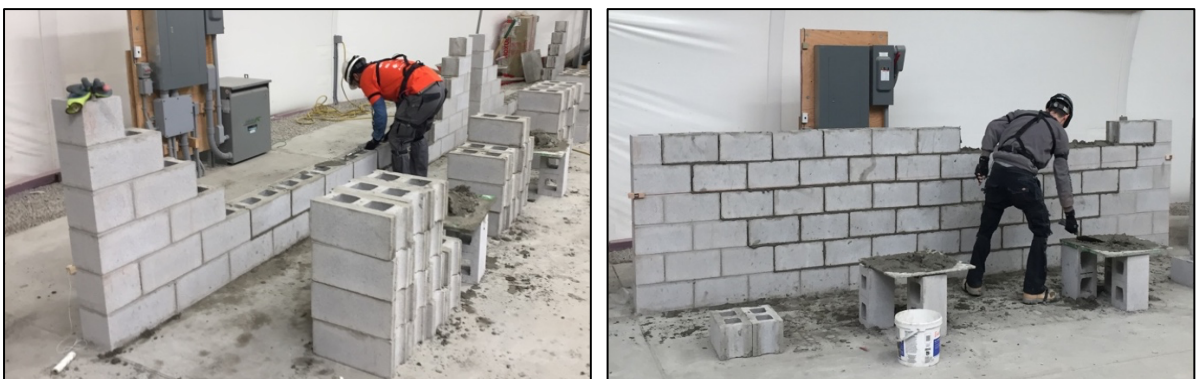
Figure 3-1: Experiment setup: placing a CMU at the 2nd course (Left), and 6th course (Right)
