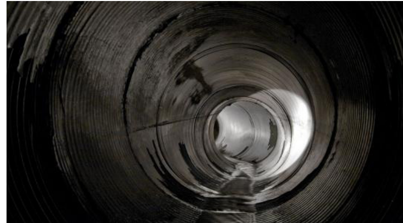
Fig. 2.1 The lost Parsons Creek of North York redirected in a corrugated metal storm sewer.
