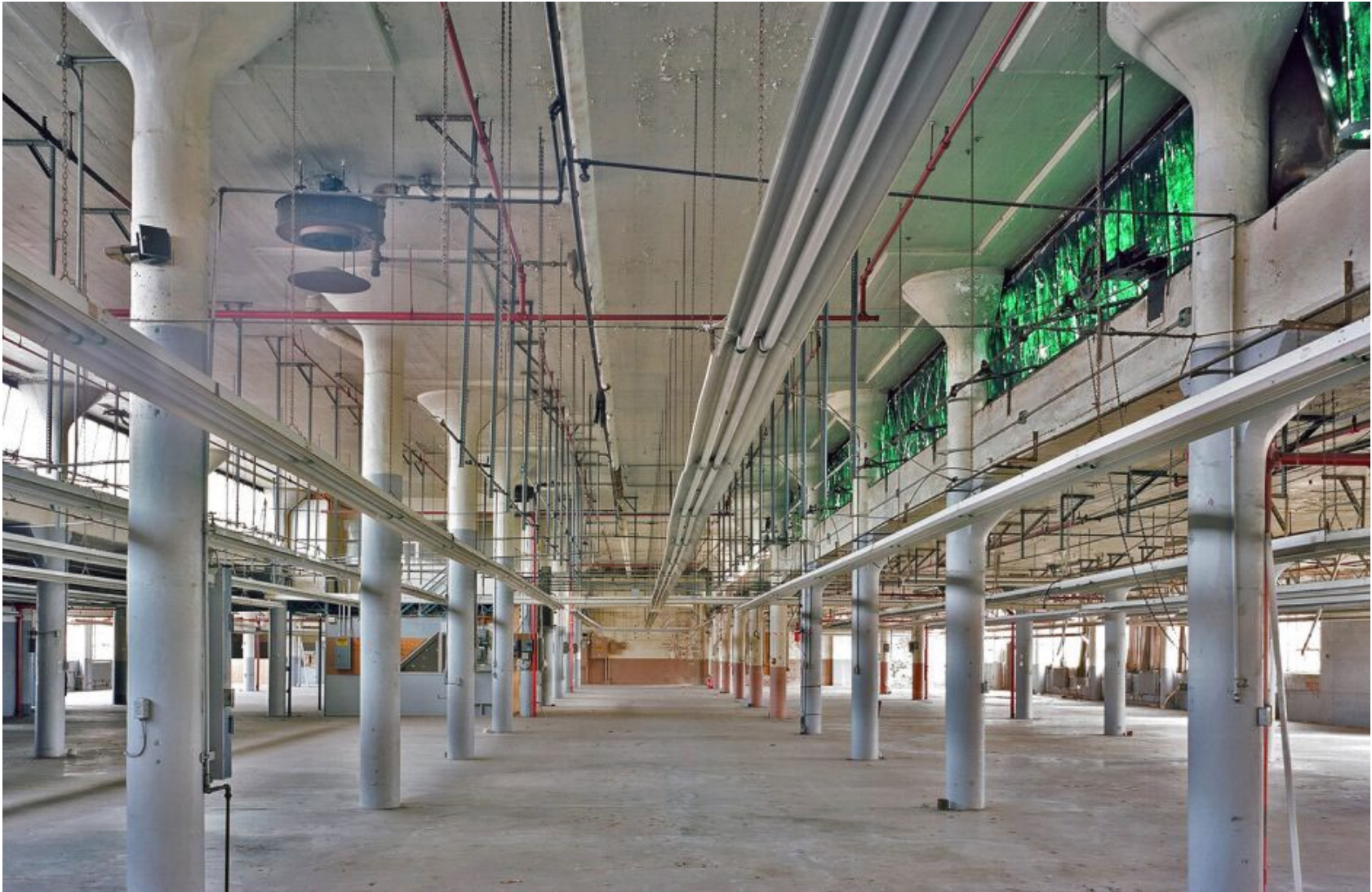
Fig. 3.14 The interior view of the abandoned Radio Stores Building.
