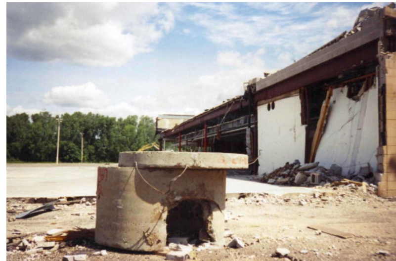
Fig. 1.7 The abandoned and deteriorating condition of Phalen Shopping mid-1990s.
