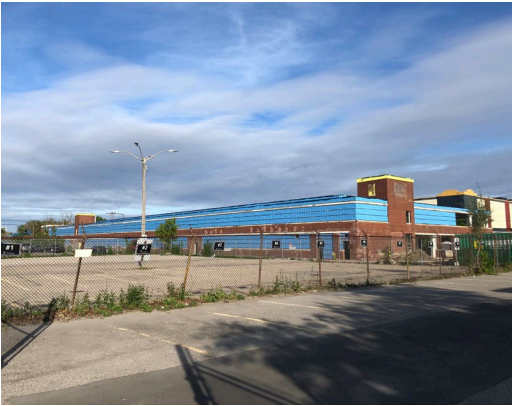
Fig. 3.1 The abandoned Radio Stores Building, Research Enterprise Ltd. and its parking lots.
