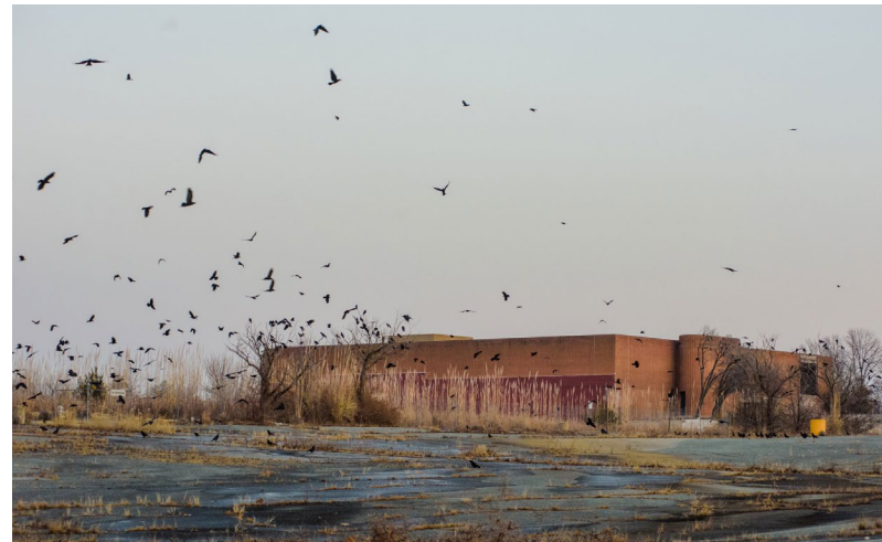
Fig. 1.4 The abandoned ruins of Landover Mall in Maryland which was taken down in 2006.
