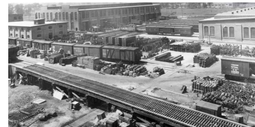
Fig. 3.5 CNoR’s railway repair building
