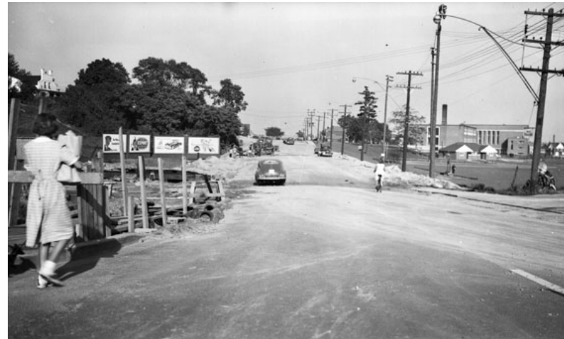
Fig. 2.22 The dip in the road (the site of the buried Walmsley brook), being 'filled in' for the construction of the new Sunnybrook Shopping Centre
