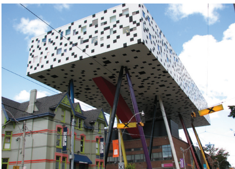
fig.0.2 The Ontario College of Art and Design Will Alsop Addition, completed 2004.
