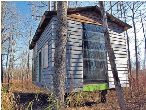
fig.4.8 Installation projects at Don Blanche.
