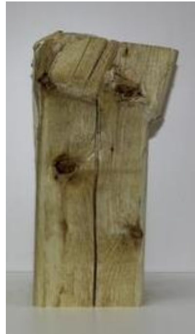
i) FRP Removed
