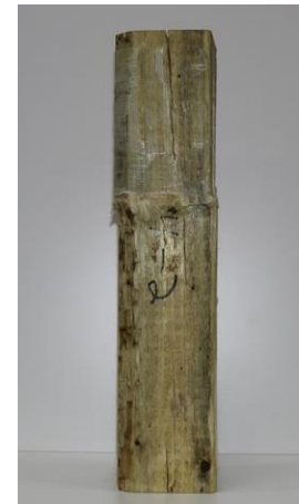
v) FRP Removed
