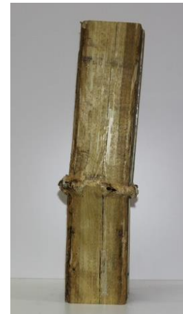
v) FRP Removed
