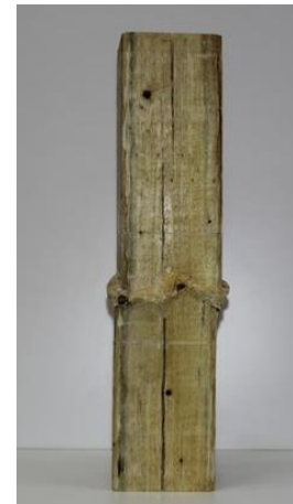
v) FRP Removed
