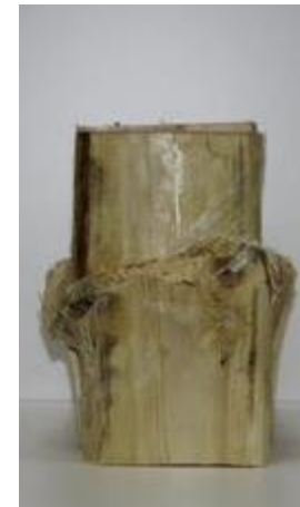
v) FRP Removed
