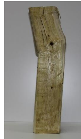
v) FRP Removed
