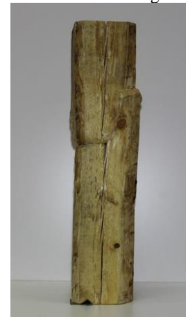
v) FRP Removed
