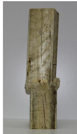
v) FRP Removed
