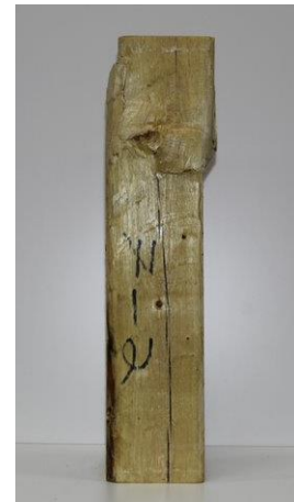
v) FRP Removed
