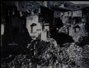
52.13 Destroyed Homes in Kessab, K1988.011.176
