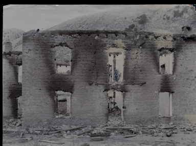
52.15 Burned American Mission Residence in Kessab, K1988.011.199
