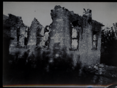
52.10 Destroyed Home in Kessab, K1988.011.171
