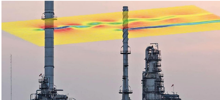
Figure 1.1. Helical strakes on smoke towers for the mitigation of VIV [6].
