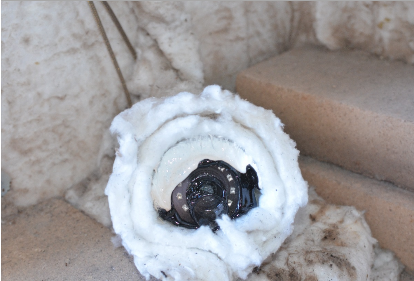
Figure 4.4: Photo showing damage to CAM1 from fire compartment conditions during Test 2
