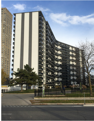
[Fig.41] 79 Thorncliffe Park Dr. existing building.
