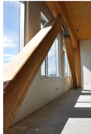
b.) University of British Columbia Earth Sciences Building Chevron BTF (Equilibrium Consulting, 2013)
