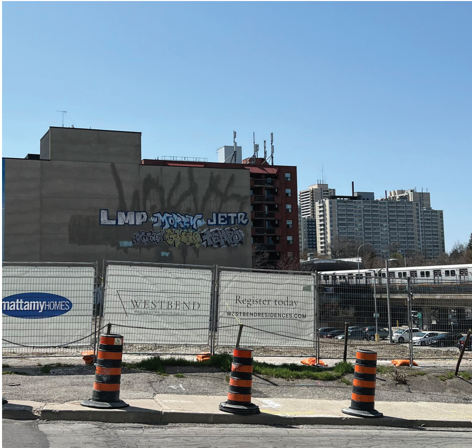
Fig. 3.17 (Above) Former location of Keele Wall, now a Mattamy Homes construction site, 2022
