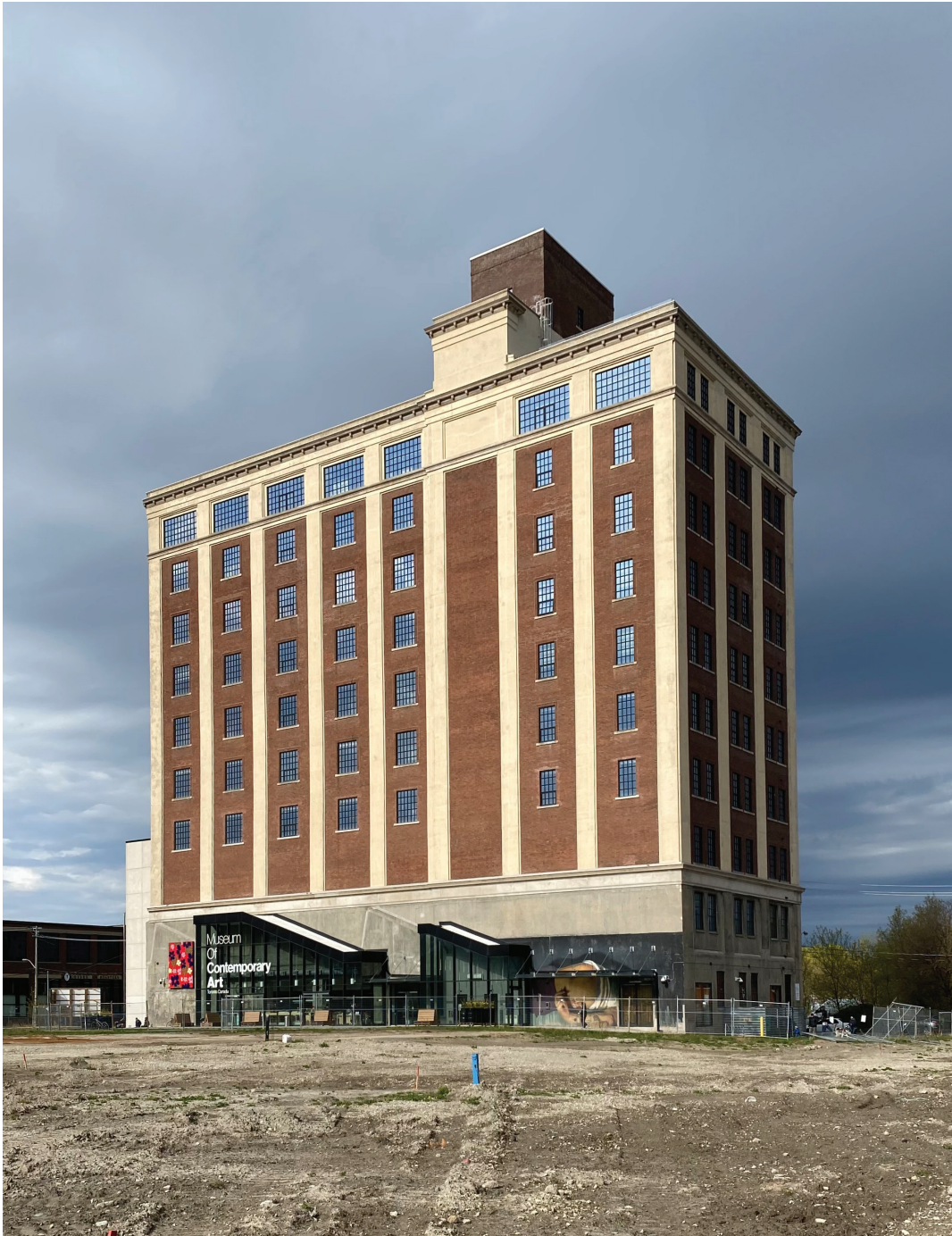
Fig. 3.4 Museum of Contemporary Art Toronto, formerly Tower Automotive Building. West facade, 2021
