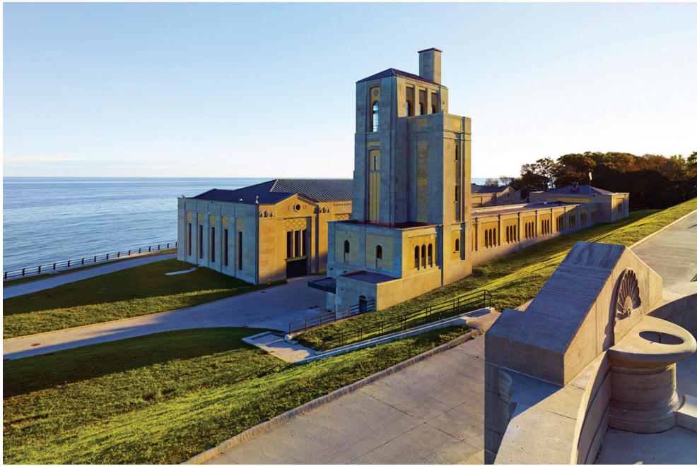
Fig. 3.15 R.C. Harris Water Treatment Plant. (Photo: Taylor Hazell Architects)
