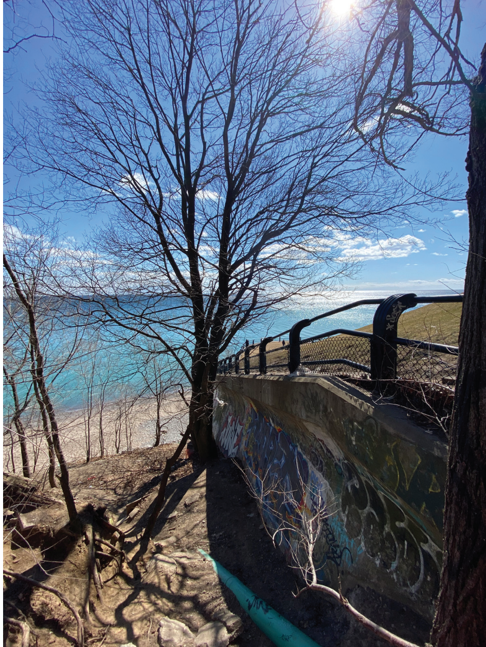
Fig. 3.16 Beach adjacent to the R.C. Harris Water Treatment Plant, 2021. Graffiti covers the retaining wall marking the edge of what I call the “underbelly” of this large and finely manicured architectural site.
