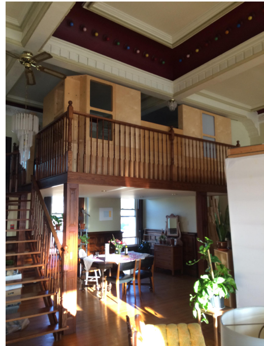
Figure 5.10 (opposite) - Disassembling one of the “boxes” to reassemble in the mezzanine
