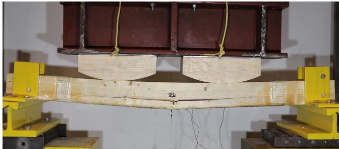
(3) Wood tensile failure near midspan
