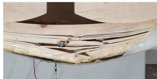
(b) Close-up of splintering damage for R9-02
