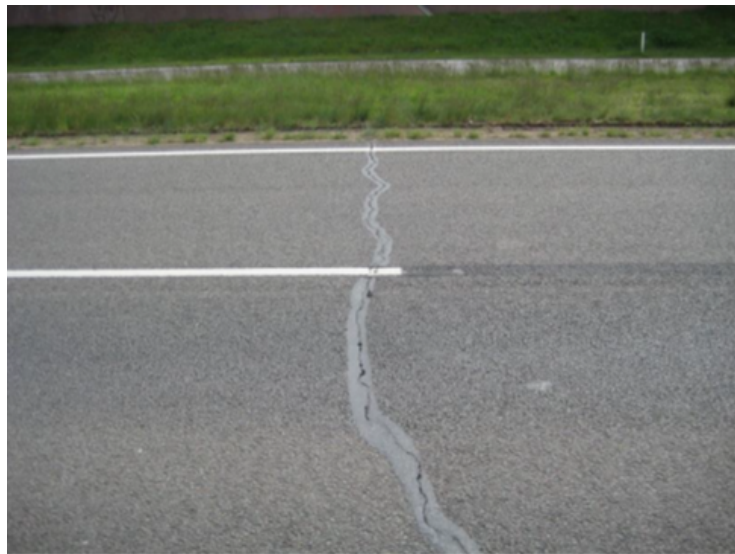
Figure 2.5: Low-temperature (thermal) cracking
