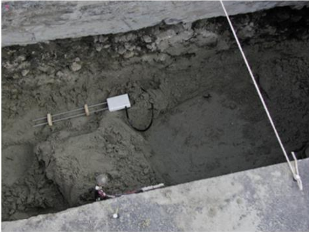
Figure 2-7 In-situ water content reflectometer (Maadani, 2015)
