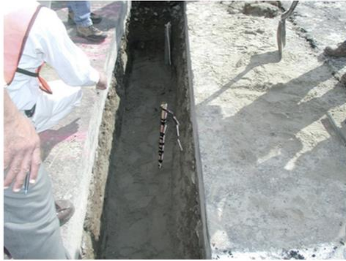
Figure 2-6 Thermocouple installation (Maadani, 2015)
