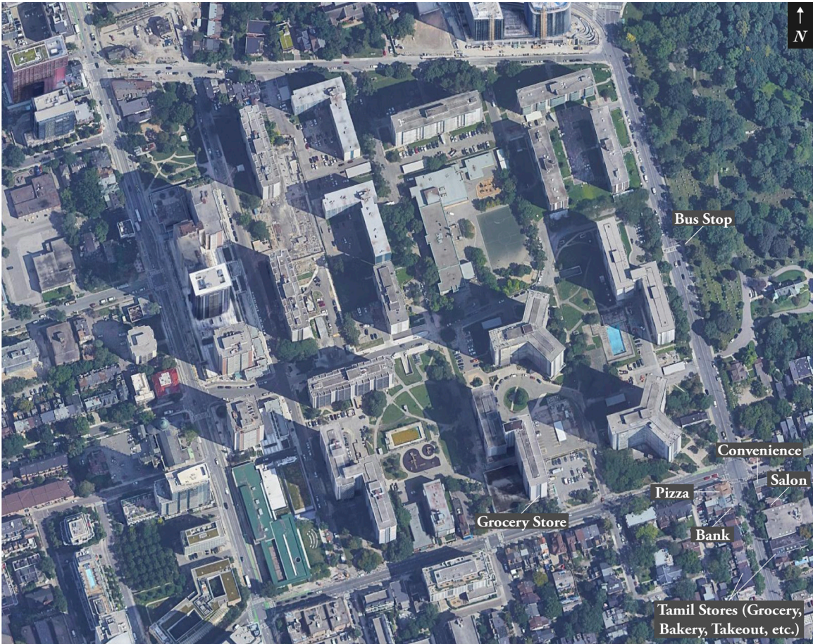
Fig. 2.1. Aerial view of the St. James Town neighbourhood, characterized by a 'tower-in-the-park' urban morphology.
