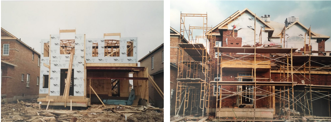
Fig. 2.10. The Milton house under construction from 2000 to 2001.
