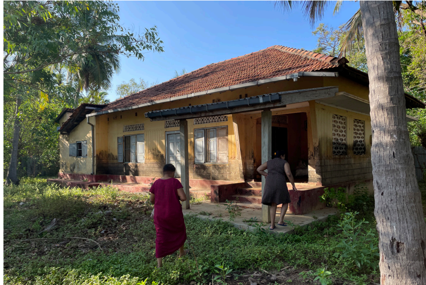
Fig. 1.3. My aunt and sibling approaching the house, constructed from 1965-68 with concrete-block walls, red cement floors, and a timber roof with clay shingles.
