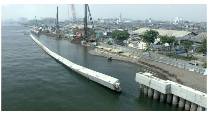
Fig. 2.13 The sea wall collapsing into the Java Sea.
