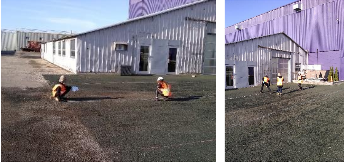
Figure 28 Site preparation for testing according to plan
