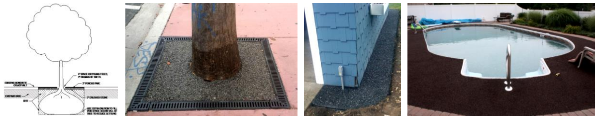
Figure 15 Construction of PRP surface in a tree well and for other uses
