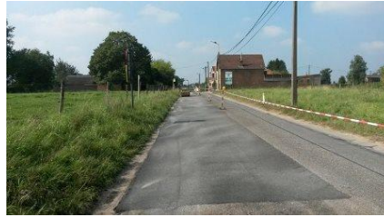
(b) Test track in Herzele, Belgium, built in September 2014 (length 40 m)
