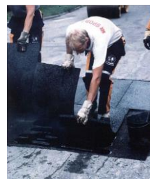
(c) Panels of PERS on the street in Sweden were laid in 1987 for winter durability testing
