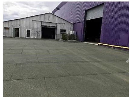
(b) Front view of the site driveway after construction
