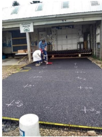
Figure 98 Site B right after construction
