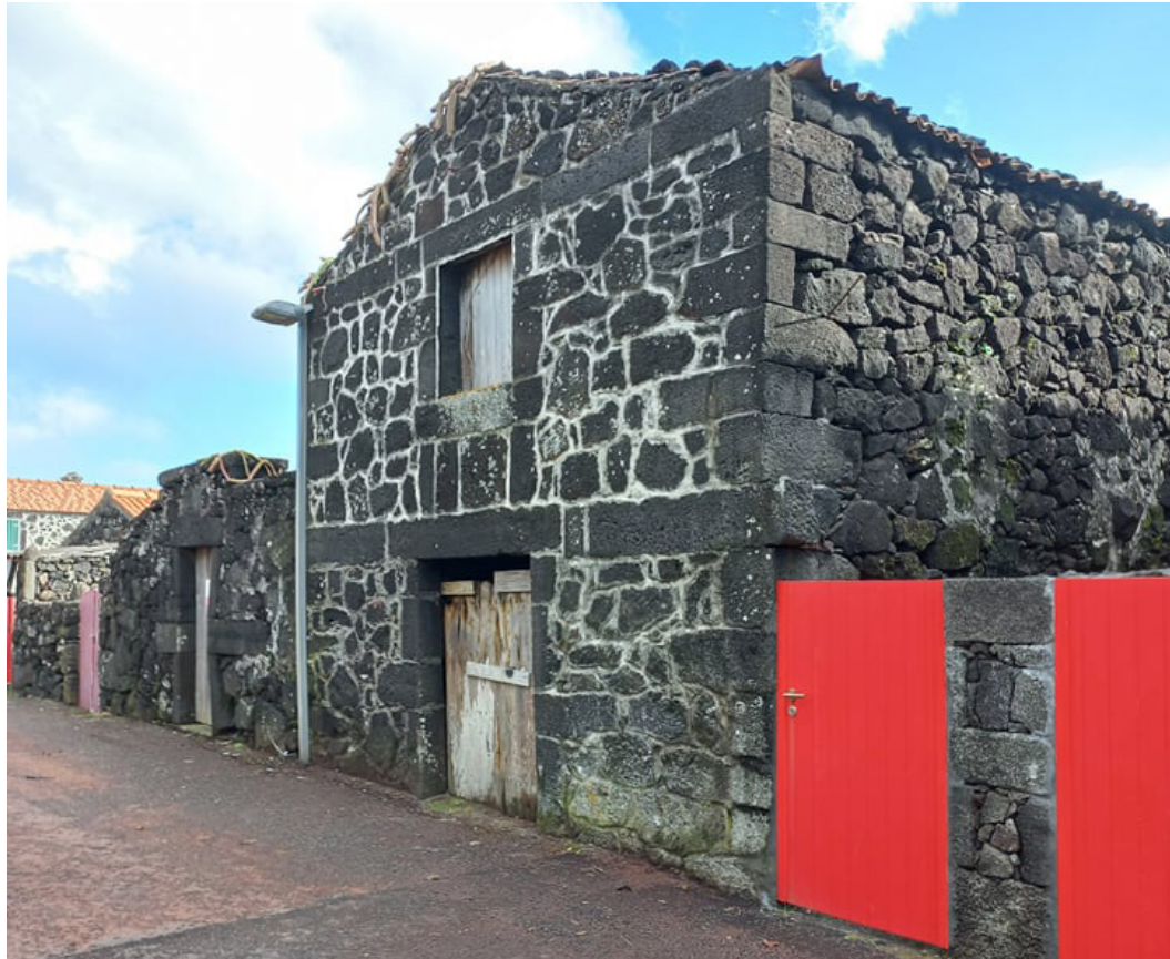
Figure 3.9: 2 floor celler considered to be without dissonance
