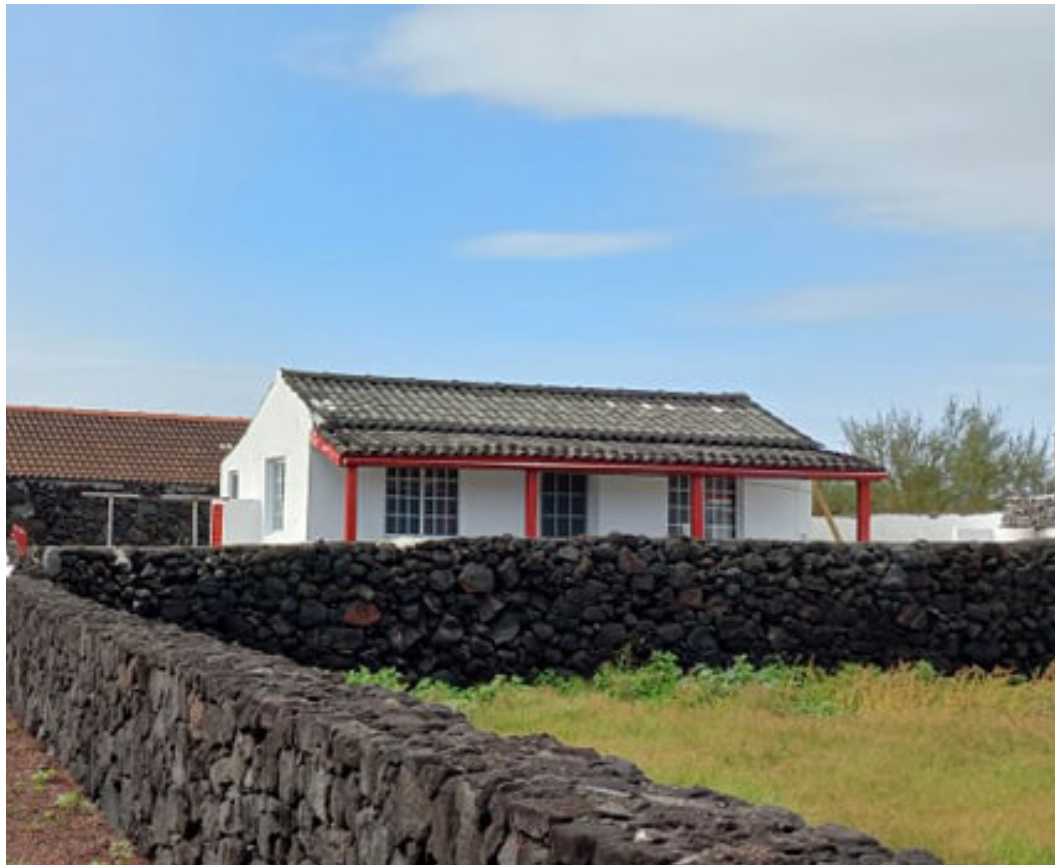
Figure 3.16: New concrete structure modern home built at the scale of traditional architecture with porch considered less significantly dissonant
