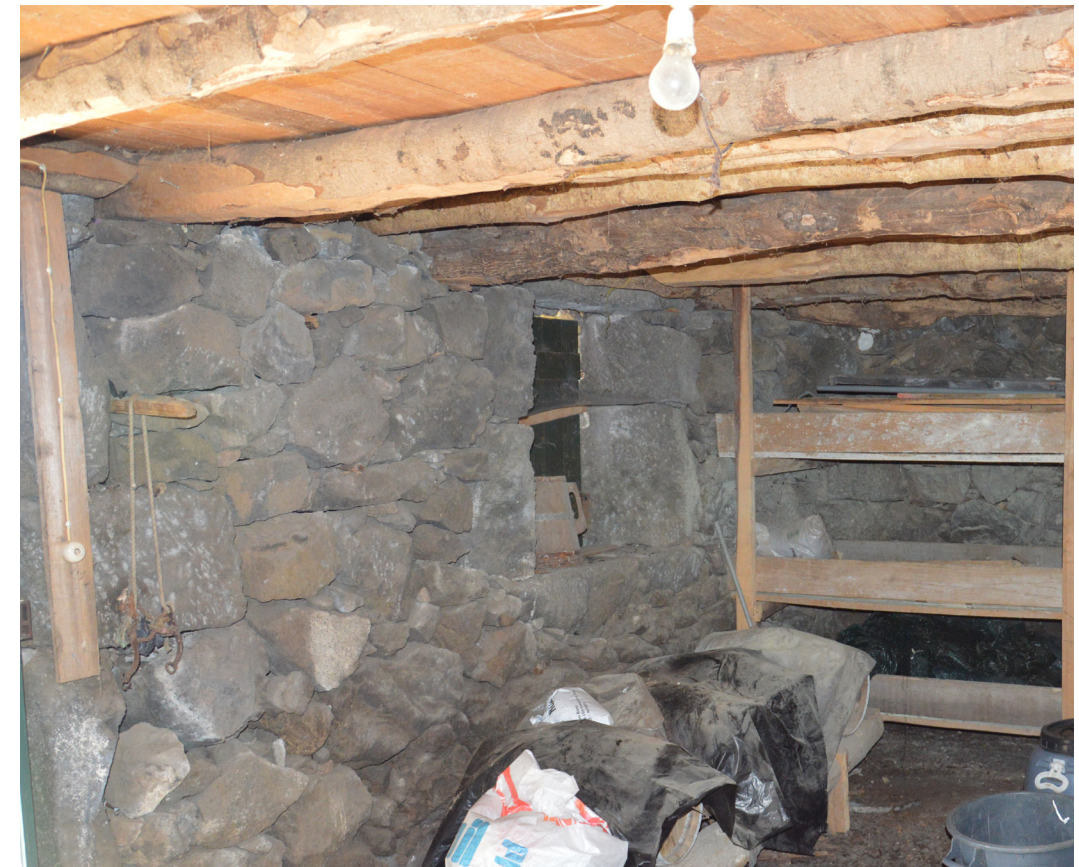
Figure 2.12: Beams in a traditional home
