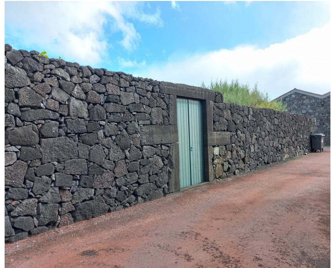
Figure 4.5: West elevation outside the wall
