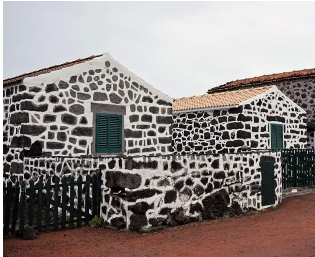
Figure 3.14: Renovated cellars that likely use some concrete considered less significantly dissonant
