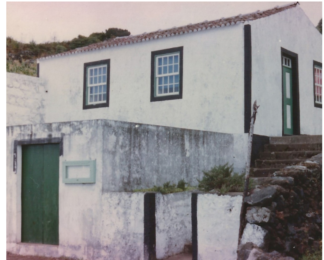
Figure 2.19: Cistern in front of home
