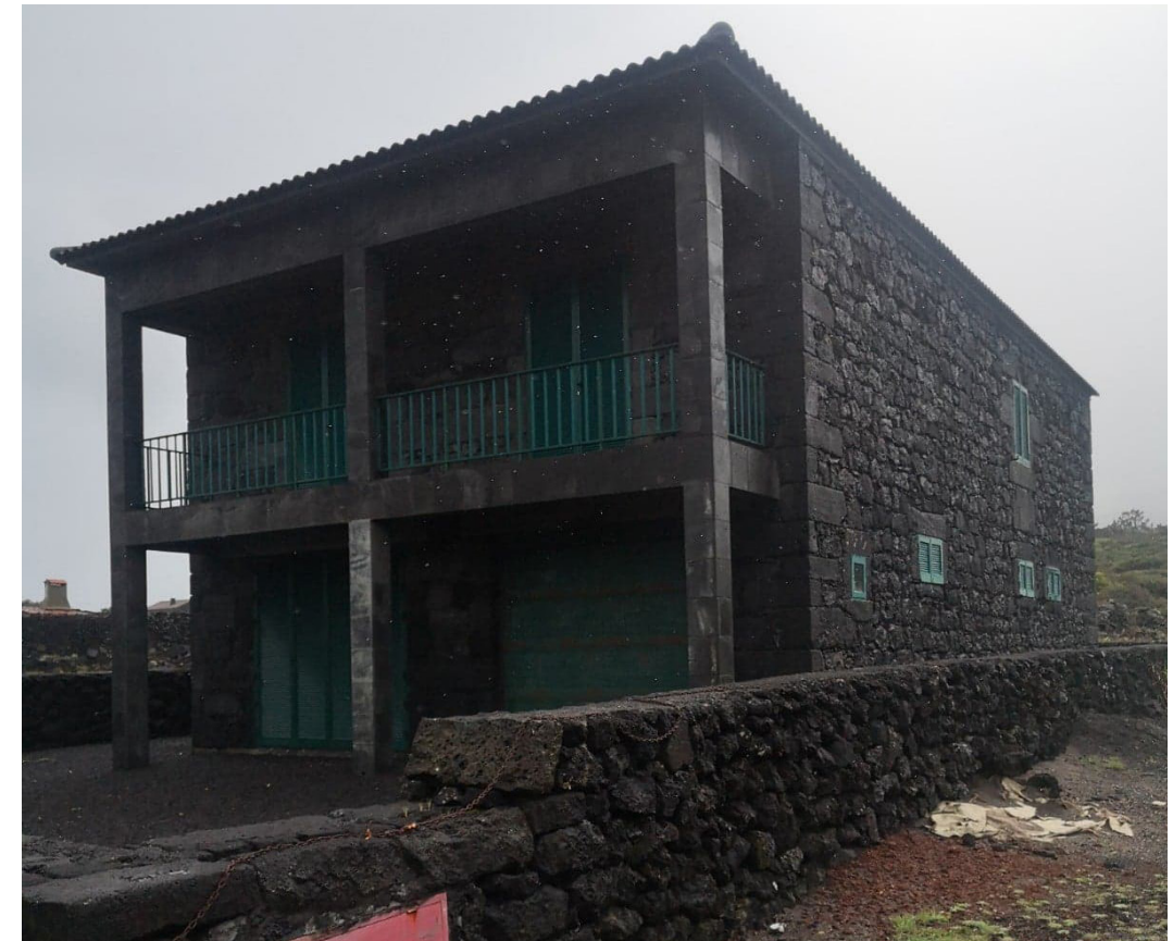
Figure 3.15: New home built with terraces, at a large scale with the potential use of a concrete frame and stone cladding considered less significantly dissonant
