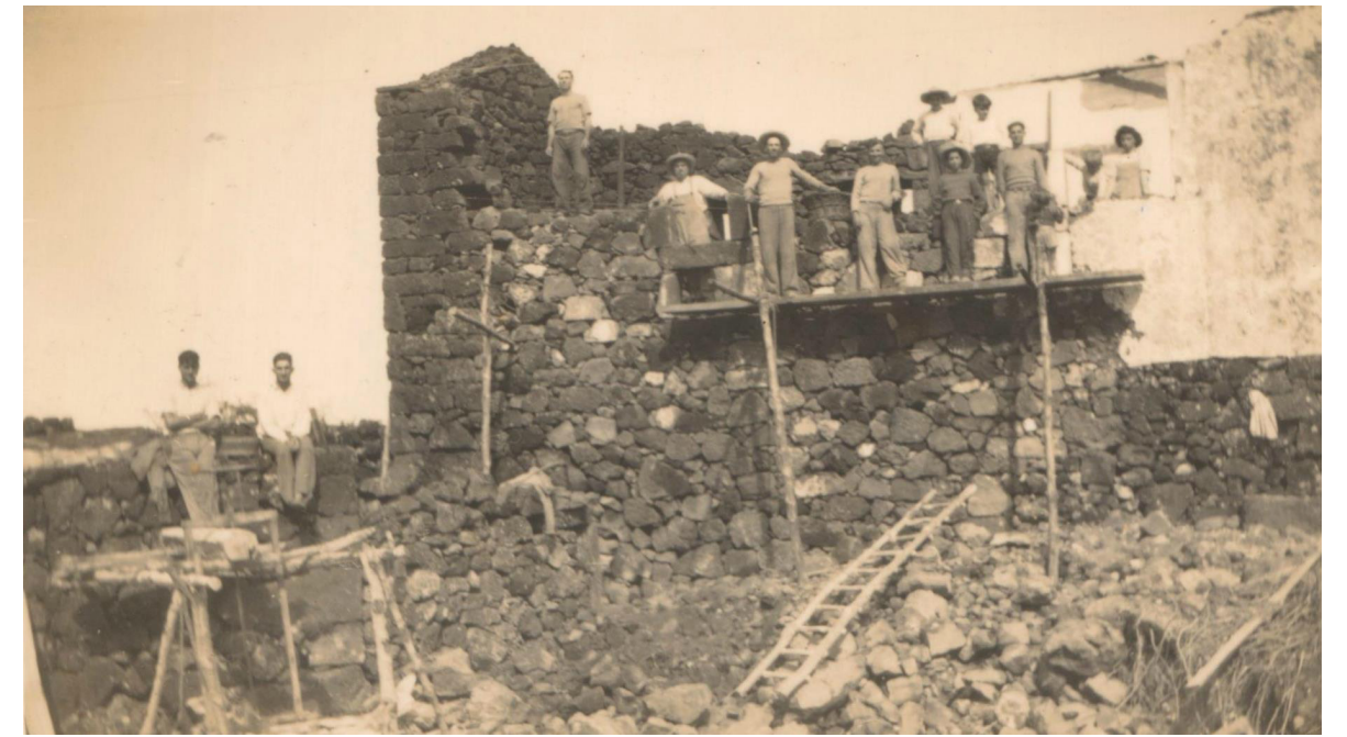
Figure 2.10: Construction Crew building traditional home
