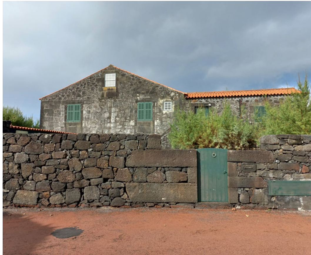
Figure 4.2: View from road
