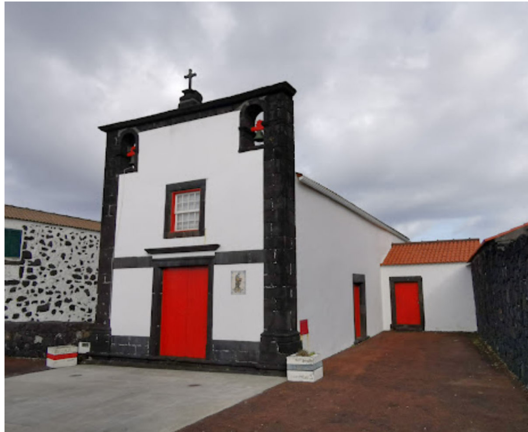
Figure 2.22: Single Room Village Chapel in the village of laijdo
