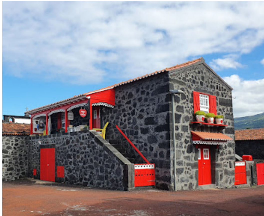
Figure 2.40: Renovation of Cellar
