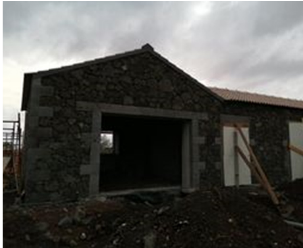
Figure 2.38: New Stone Wall with Grey endstones
