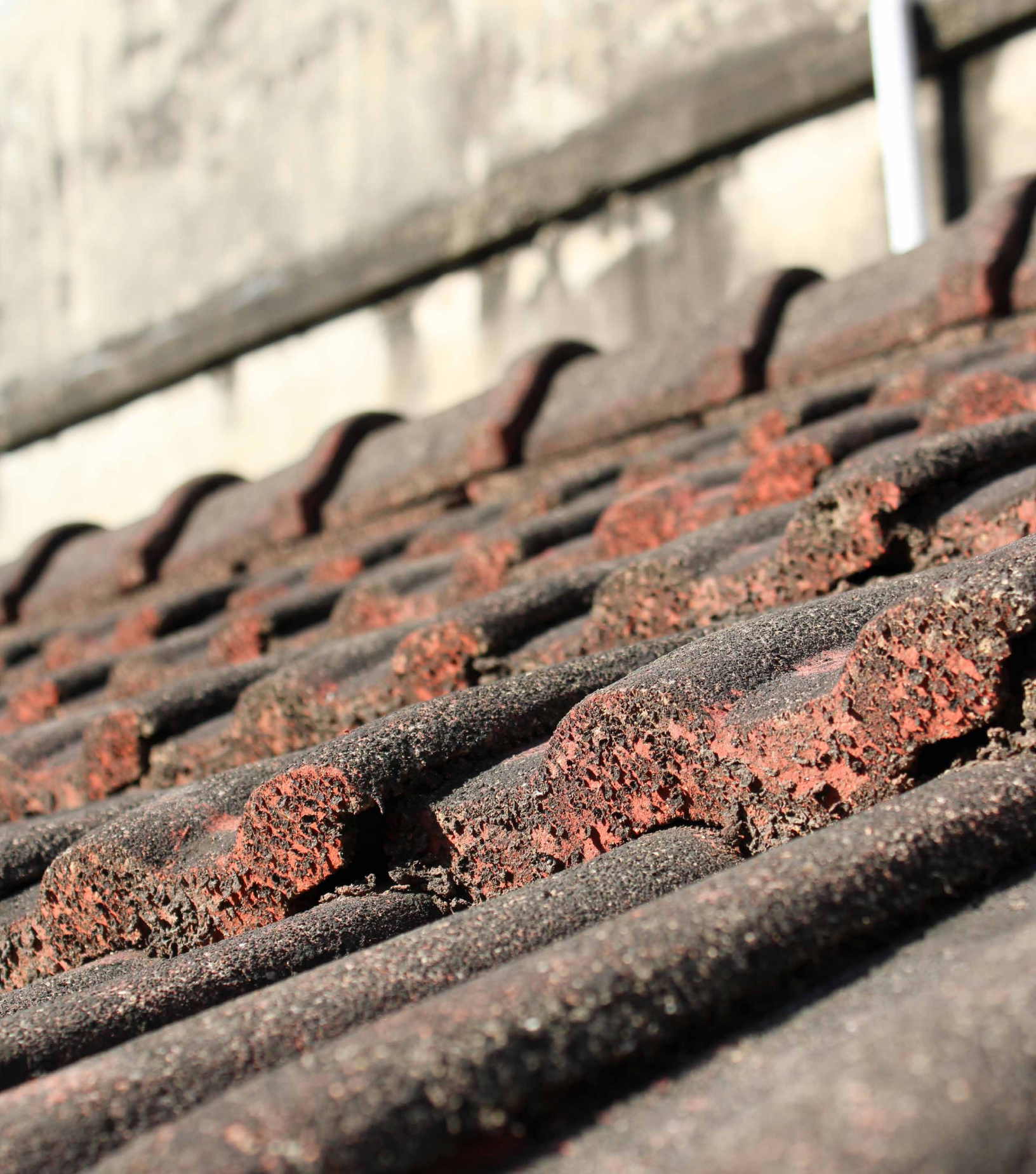
Fig. 6.88 A Traditional Chinese terracotta roof. Terracotta tiles have been used as early as 771 BC in Chinese culture and has been a common material in Tainan ever since the integration of the Han Chinese and Dutch colonies in the 17th century. The seemingly black coating and texture on the tiles is due to years of moss growth and flaking 48 .
