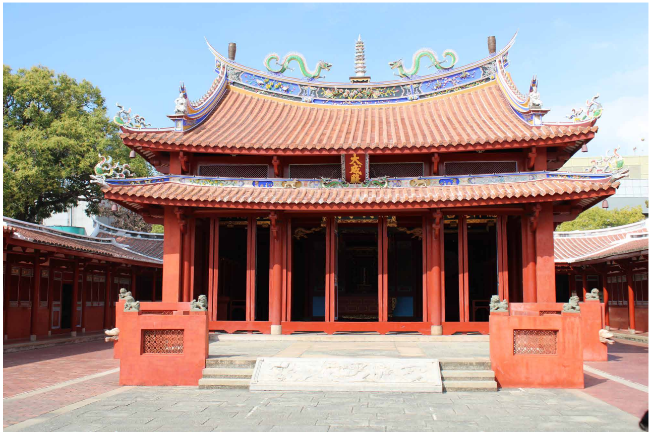
Fig. 2.32 The Confucius temple located in Tainan, which also doubled as the first established school in Taiwan. Note the temple's resemblance to the Minnan-style home with a swallowtail roof and symmetrical layout
