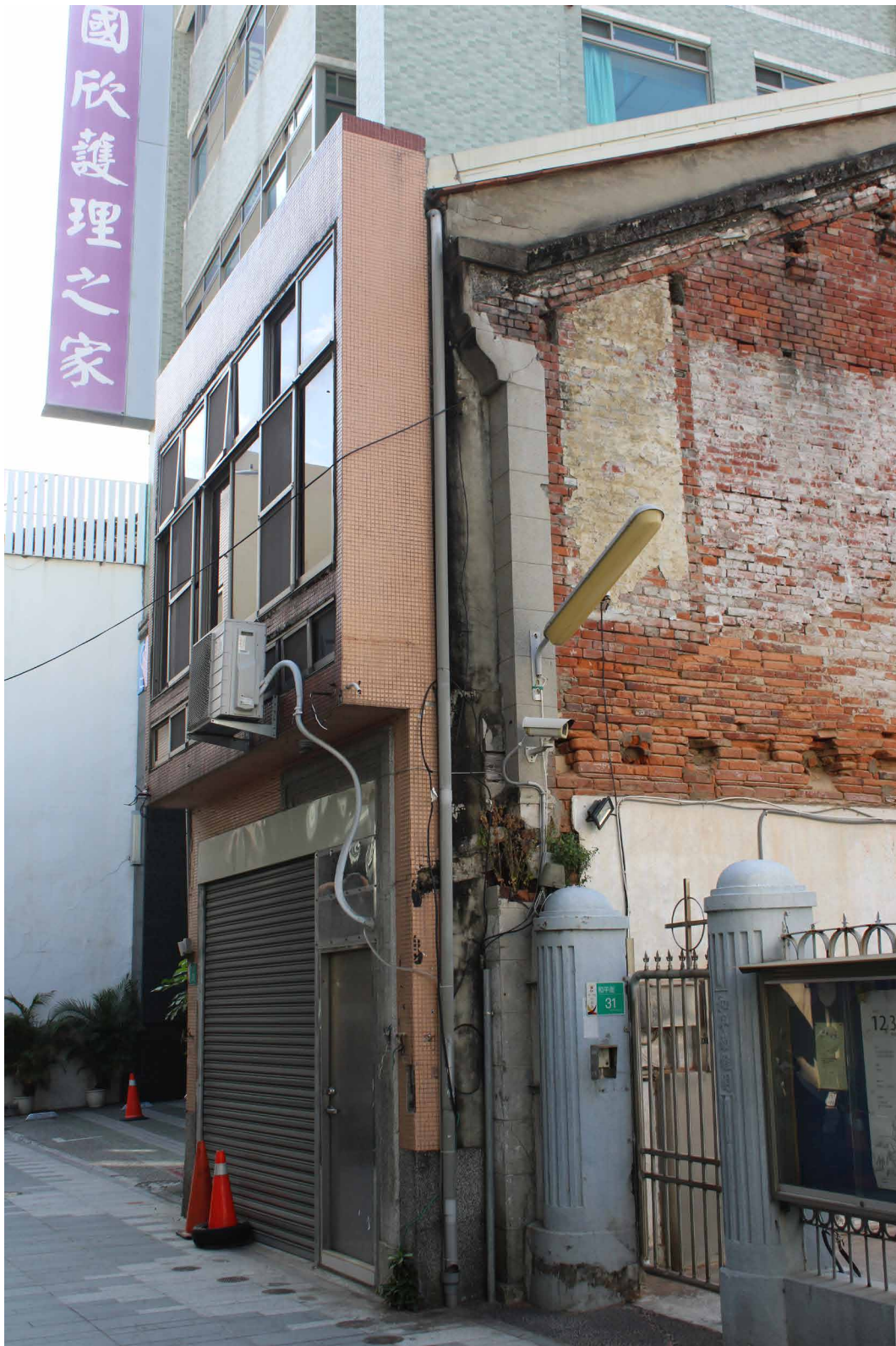
Fig.0. 12 A traditional masonry home with a modern facade attached to it, which was likely a result of the residents only remodeling a portion of their home.
