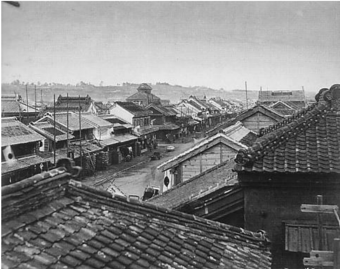
Fig. 3.56 A row of traditional Machiya streethouses from the Meiji Era of Japan. This type of building consists of solid rows of houses all facing the same direction. The Machiya House is traditionally made out of wood but houses built during and after the Japanese Showa era can also be made of materials such as masonry, concrete, and plaster.
