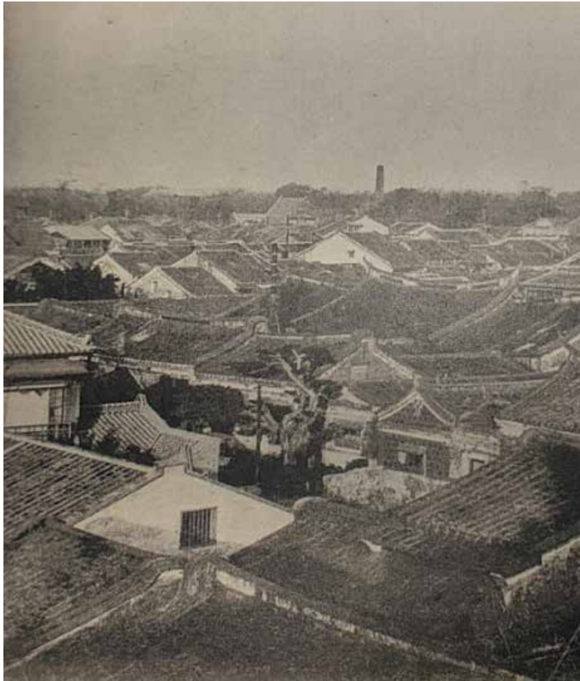
Fig. 2.30 Postcard from 1901 shows a traditional Minnan-style neighborhood which has yellow pointed tips and a curved roof surface. Regular residential buildings have horseback roofs also highlighted with swallowtail roofs but are adorned with
