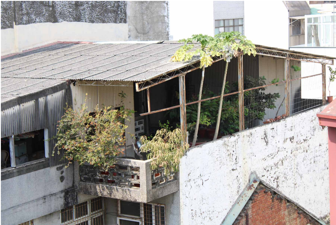
Fig. 2.53 A rooftop space made of steel decking that is used as a garden space by the resident.
