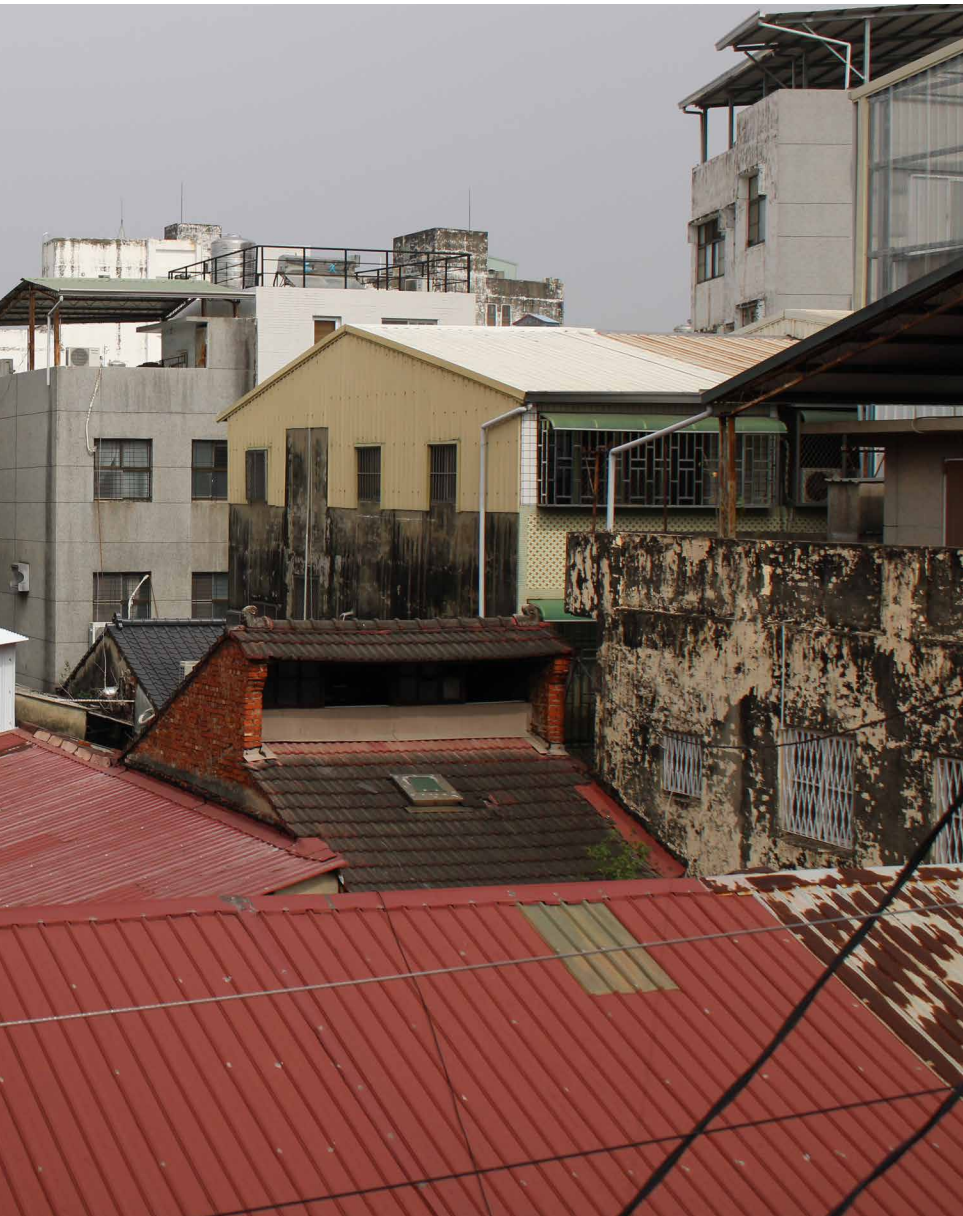
ne and form a microcosm of different cultures within the neighborhood. Traditional nt additions of corrugated metal roofs and balcony spaces. A modern mimic of the hidden behind one of the Chinese homes. (center of photo)
