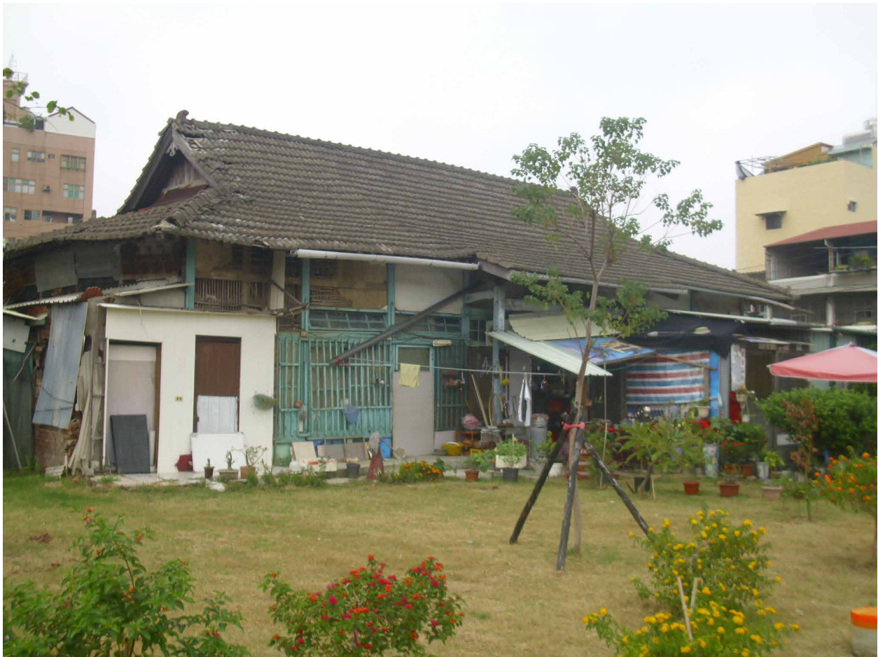
Fig. 3.562 A home that has experienced quite a heavy amount of modifications by its residents. The house seemed to have originated from the Japanese colonial era, as the roof is constructed in a distinct Japanese style called the Irimoya style, and some of the original wooden structures can still be spotted on the house.
