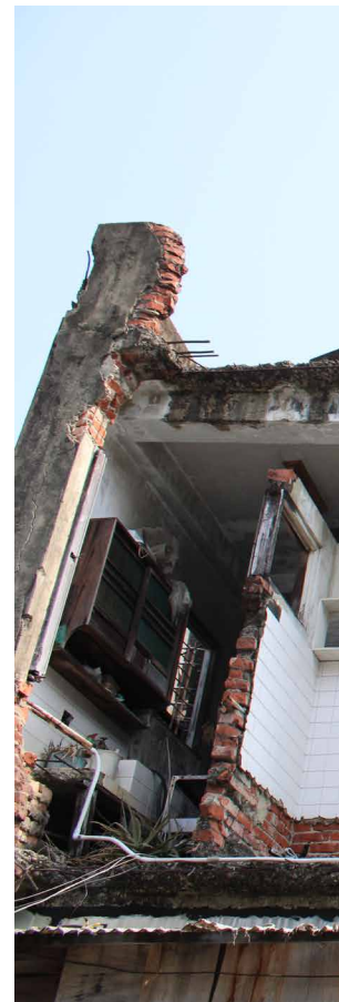
Fig. 7.124 (left) - 7.125 (right) A roadside home that was abandoned with one of its walls missing, allowing one to see the history of the house clearly. One can see a clear distinction of the original structure (judging from the cupboards and tiles), and the concrete structure added later.
