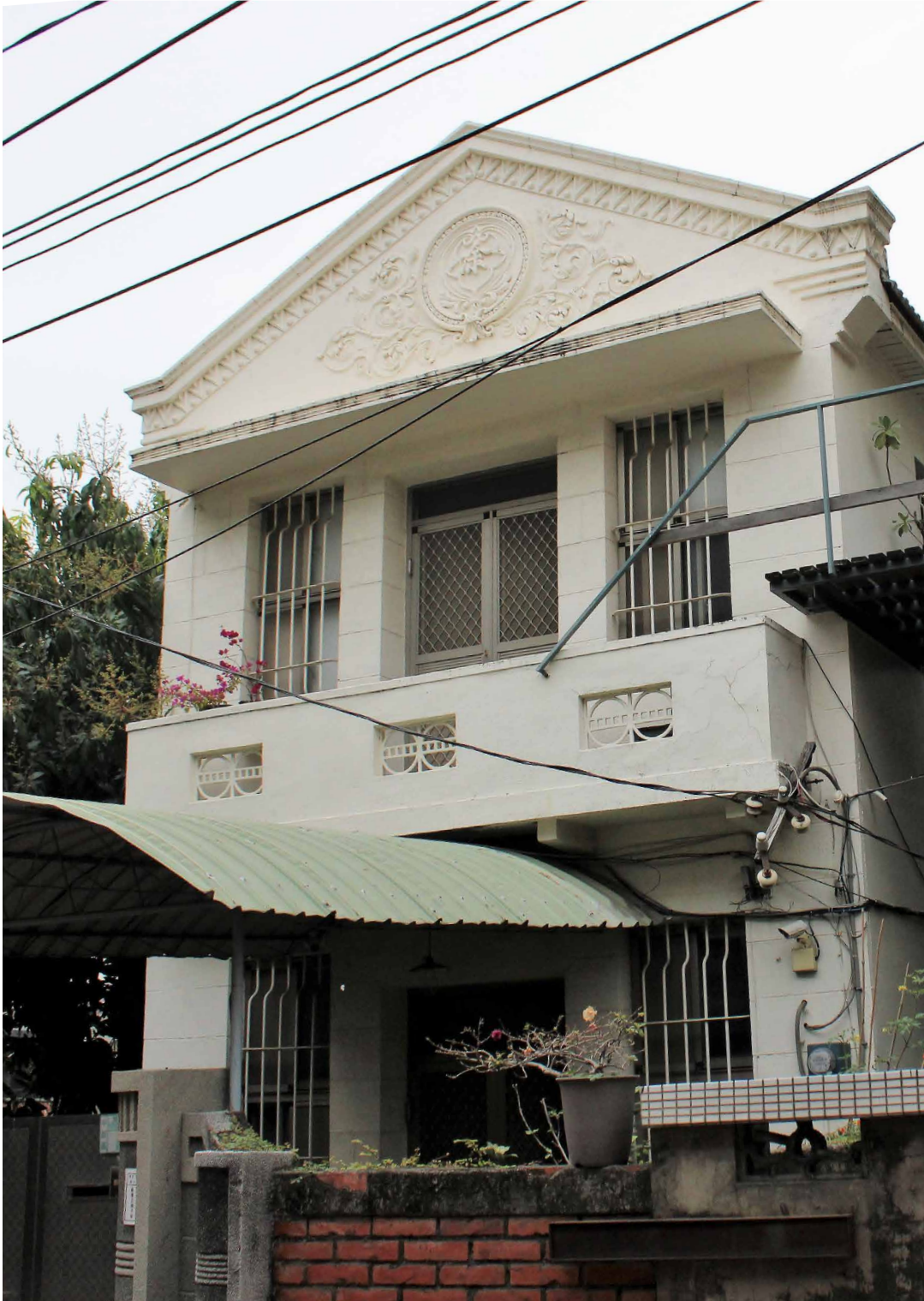
Fig. 2.41 A Japanese colonial house in Tainan. This Showa style home, adorned with a family crest on the roof, was likely owned by a wealthy official working for the Japanese Army as they were typically given better treatments than the rest of the population.
