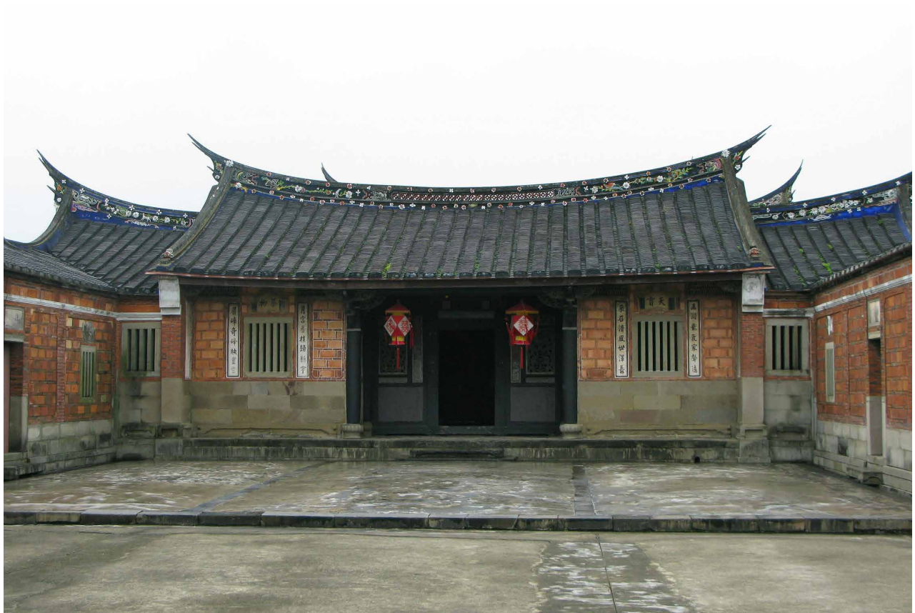
Fig. 2.31 A Traditional Minnan-style ancestral hall within a courtyard typology home. These homes are built to resemble temples with symmetrical architecture and terracotta roofs. This particular roof style is called a swallowtail roof. Depending on the region and status of the residents, some homes will have ornamented roof ridges, as is the case with this particular one decorated with ceramic depictions of flowers and animals.
