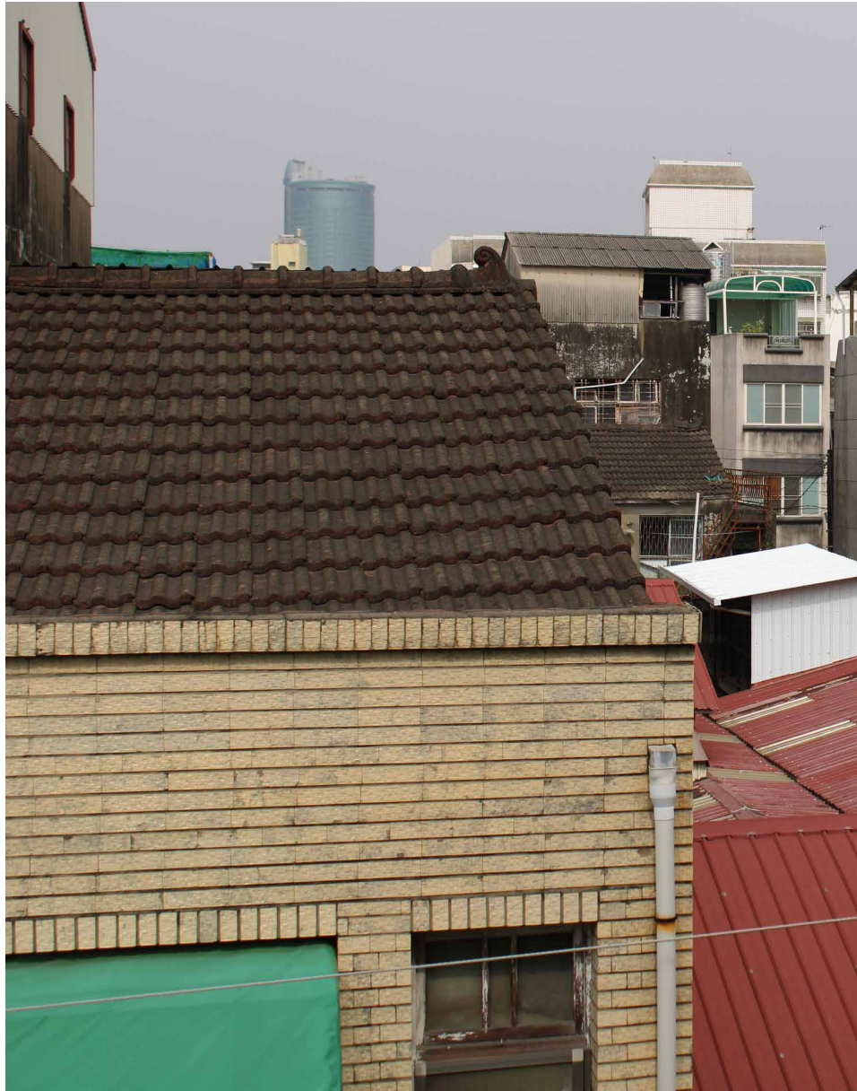
Fig. 1.20 A diverse range of roof styles and heights tell of the history of each home. Chinese terracotta roofs from the 19th century share their space with more recent Japanese kirizuma (meaning gable) roof can also be seen.
