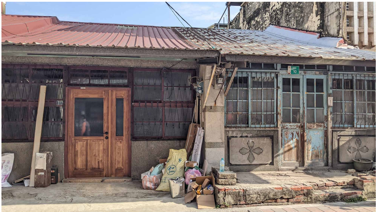
Fig. 3.63 Two homes that appeared to have undergone reconstruction at different periods of time, branched off from the same Minnan-style home according to other residents in the neighborhood. One can also identify this based on the general low-rise, linear, and symmetrical form of the house. The house on the right seemed to have been modified during the 1950s~1980s, when the floral star pattern etched on washed terrazzo and the wooden exterior were popular. The house on the left is currently under remodeling and will soon become a hair salon.
