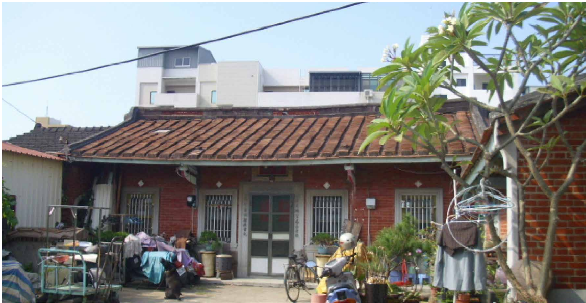
Fig 2.28 - 2.29 A well-preserved Minnan style home located on the outskirts of Tainan, which still retained a courtyard due to the abundance of space in rural regions. One can identify these houses by looking at the its roof, construction material, or the symmetrical layout of the main entrance.
