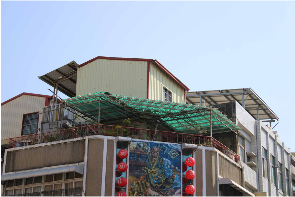
Fig. 2.52 Some colorful rooftop additions can be seen tacked onto existing building structures, creating additional open or enclosed spaces for residents to utilize.
