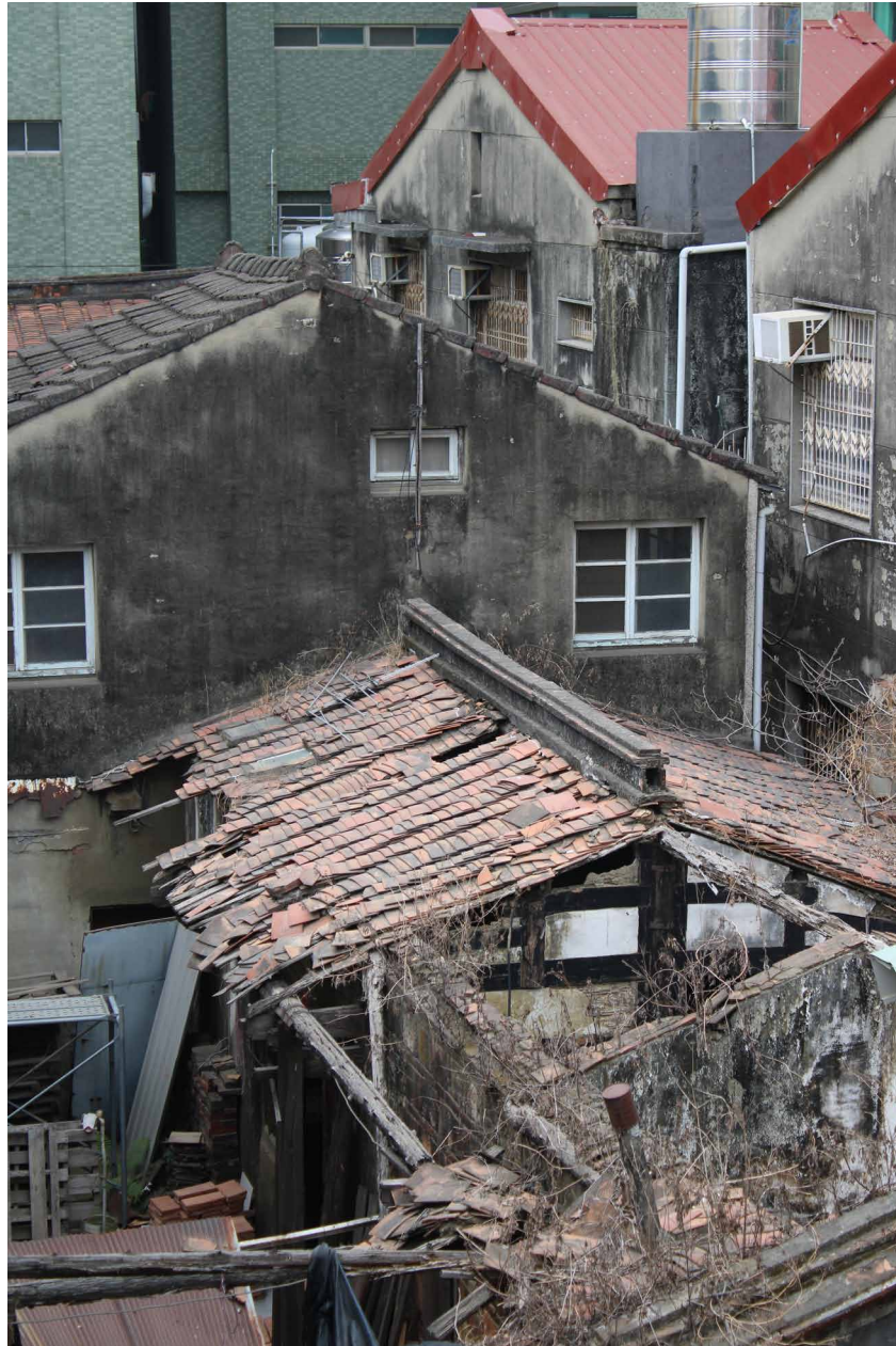
Fig. 7.119 zoomed-in photo of the previous ruins. One can see the terracotta material and wooden structure of the roof in this photo
