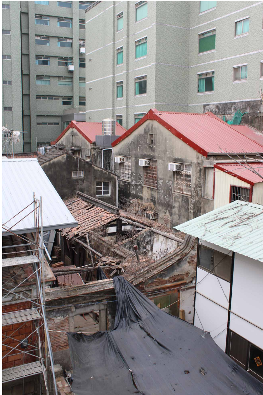
Fig. 7.118 a set of Minnan style ruins surrounded by high-rises and more modern buildings on all four side. Thankfully, one of the residents who lives in the surrounding area has informed me that a preservation project has been initiated.
