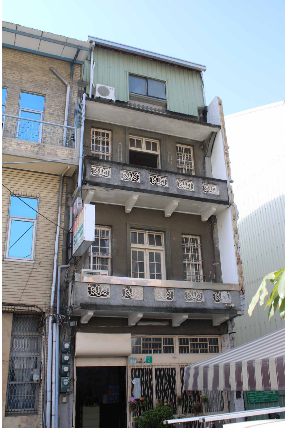
Fig. 7.111 The pharmacy owned by Ms. Tsai and her family, which also serves as their family home. The building to the right of their house has been demolished, but some parts of its walls are still attached to the pharmacy. The metal guards embedded in the balconies makes the building appear very prominent on their street. Ms. Tsai told me that the house has gone through many modifications; the door and windows on the first floor have been completely replaced at one point, and the metal decking addition on the fourth floor was also added later.
