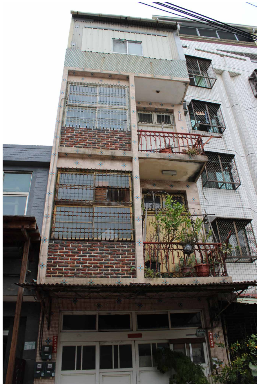
Fig. 2.48 (left) - 2.49 (right) Some examples of contemporary homes in Tainan. The manufacturing processes and abundant imports of various materials and ornaments allow used brick veneers, mosaic tiles, and decorative handrails to create a colorful facade on covered with green mosaic tiles and has incorporated a space on the first floor for shops houses, which can be used as an extra enclosed room (Fig. 2
