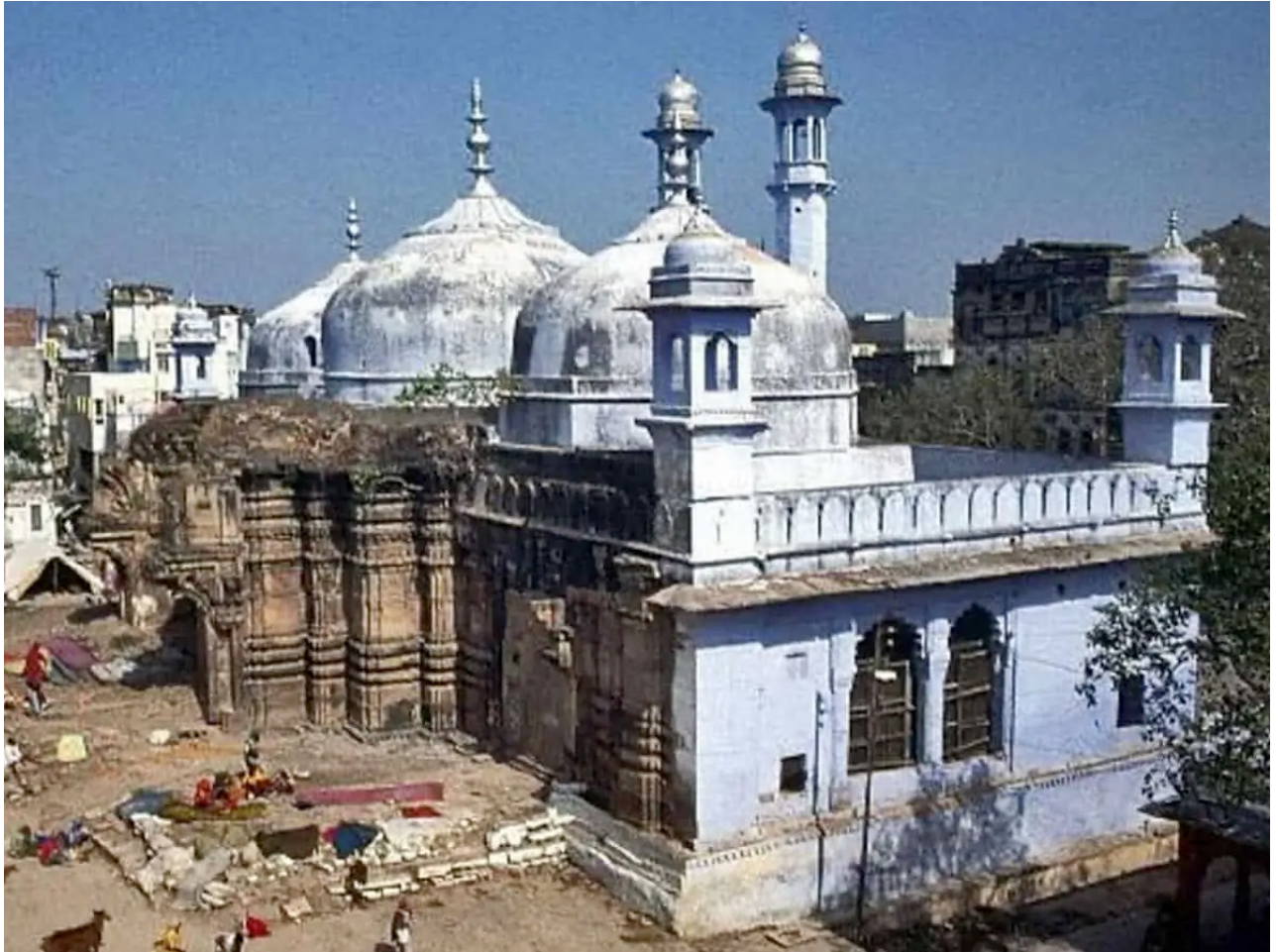
Fig. 2.2 A view of the Gyanvapi Mosque's rear wall, where remnants of an older demolished structure still remain.
