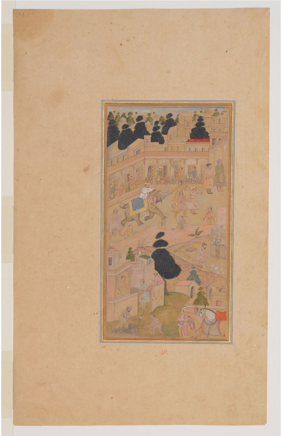
Fig. 4.2 Construction at Akbar's new capital Fatehpur Sikri, Balchand, c.1603-1605
