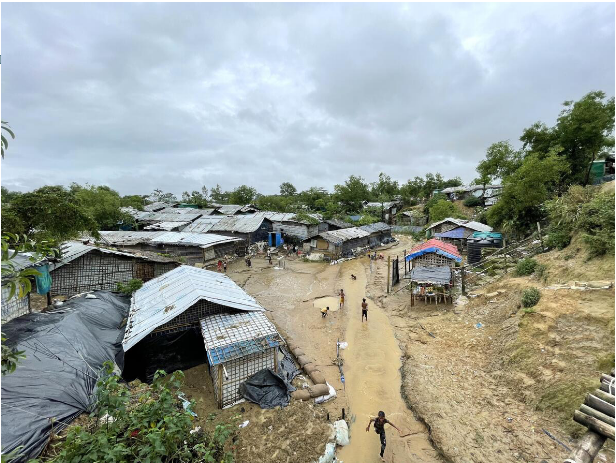
Figure. 3.14. To facilitate the need for living spaces for refugees, stairs and terraces were cut into the existing landscapes so quickly that it resulted environmental disaster such as flash floods and mudslide, 2021, Top and middle right image Source: UNHCR
