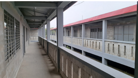
Figure. 3.30. The exterior view of the houses and the interior of bunk-bed rooms. Credit: Shamsuddin Illius/The Business Standard, 2019.
